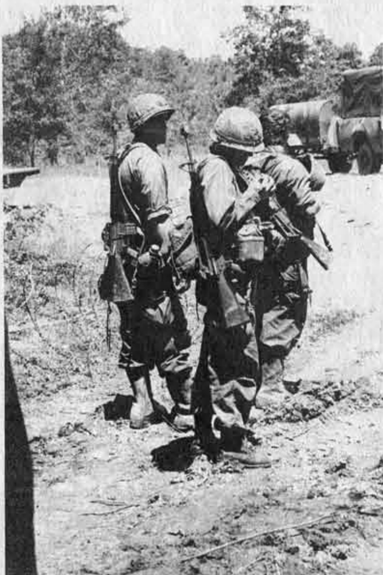
ENGINEERS AWAIT a lift to the bridge site.
