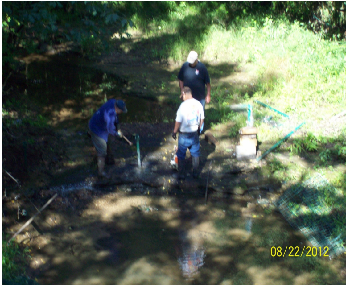
Pictures of Sand Creek Barrier During Removal 21-22 Aug 2012
