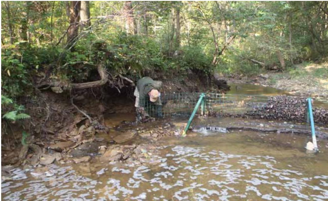
PICTURE SHOWING UXO TECHNICIAN REMOVING ACCUMULATED DEBRIS FROM BARRIER
