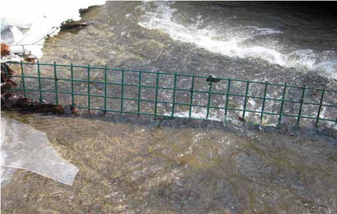
CLOSEUP OF UPSTREAM BARRIER FOLLOWING CLEANUP.
