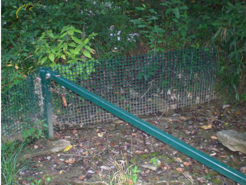
Photo 3: Downstream barrier, north end panel (2 September 2009, before O&M)
