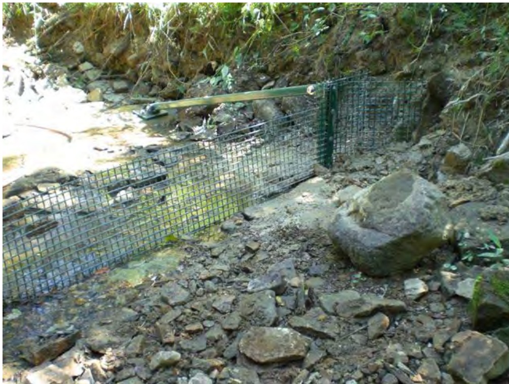
Photo 4: New post and panel at south end of downstream barrier (2 September 2009)
