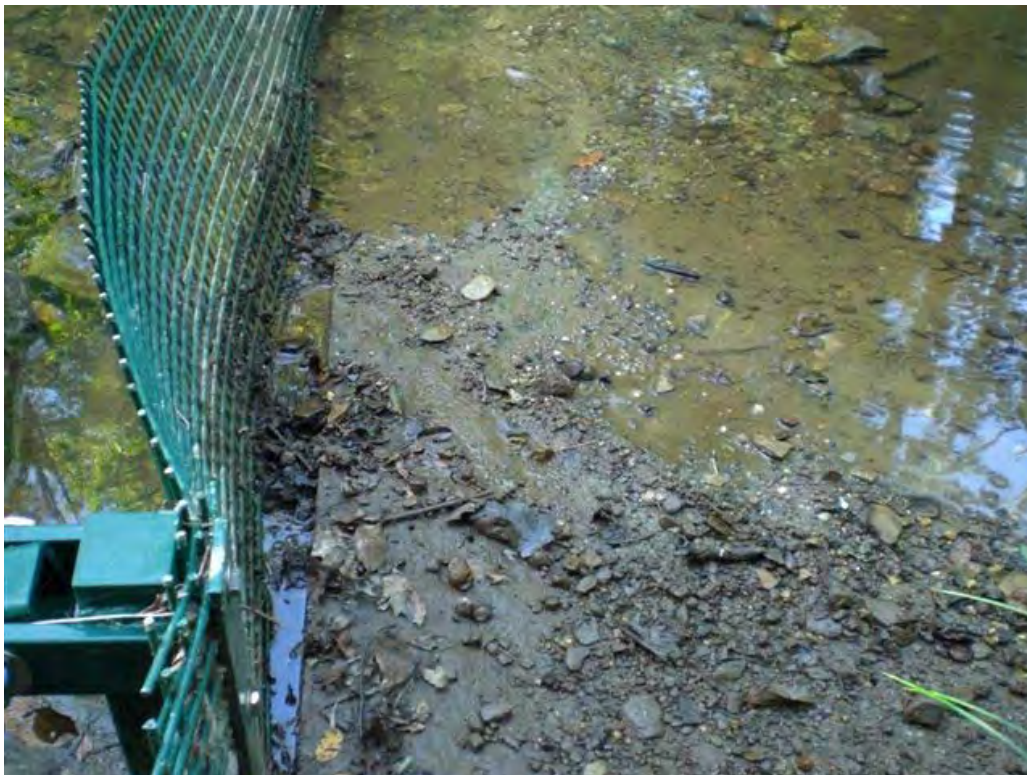
Photo 8: Area in front of downstream barrier after the removal of sand and gravel accumulation (2 September 2009)
