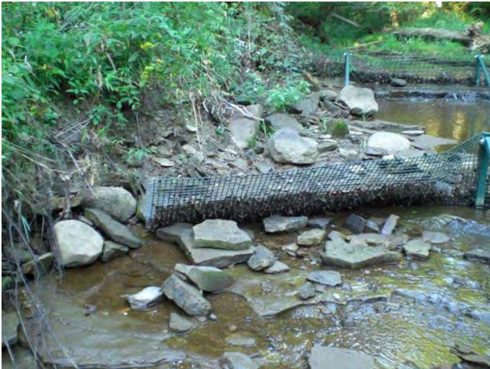
Photo 2: Downstream barrier, south end panel (2 September 2009, before O&M)
