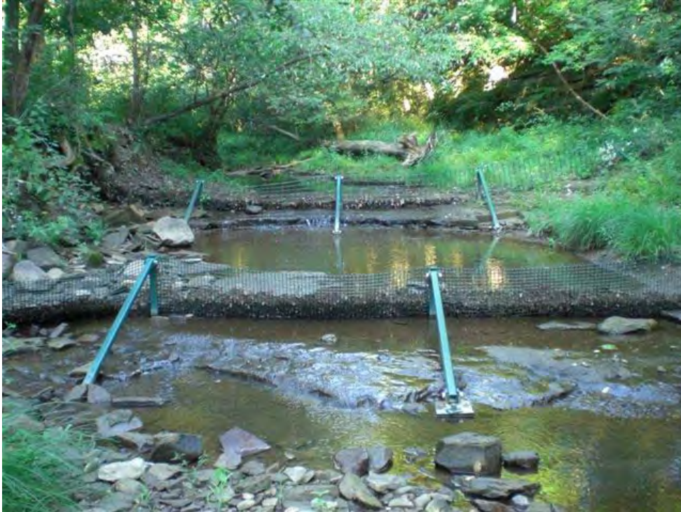
Photo 1: Sand Creek Barrier System (2 September 2009, before O&M)
