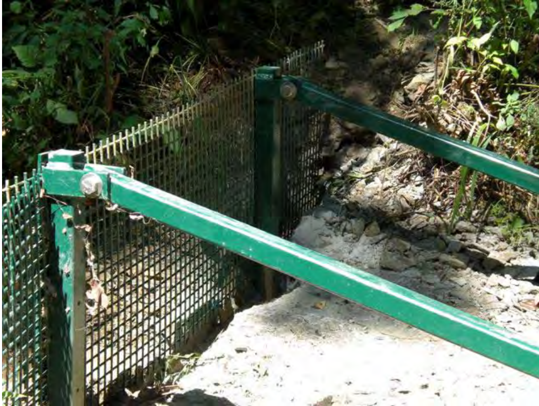
Photo 5: New post at north end of downstream barrier (2 September 2009)
