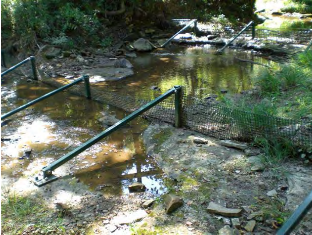
Photo 7: Downstream panels after height reduction (2 September 2009)
