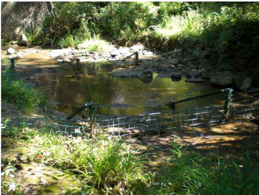
Photo 6: Upstream panels after height reduction (2 September 2009)
