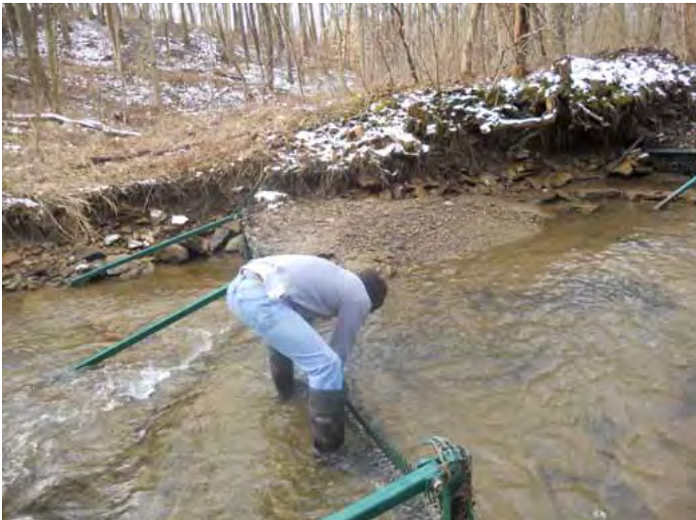
PICTURE SHOWING UXO TECHNICIAN REMOVING DEBRIS FROM BARRIER.
