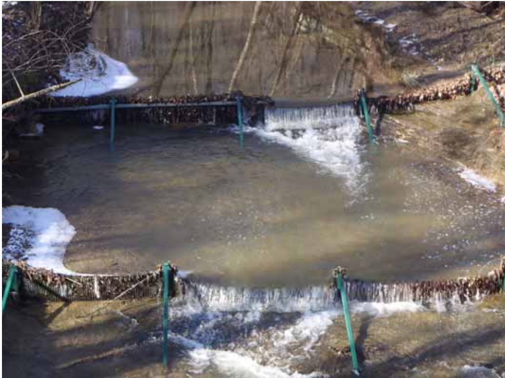
PICTURE SHOWING BUILD UP OF SAND AND ROCK ON SOUTHERN END OF BARRIERS.
