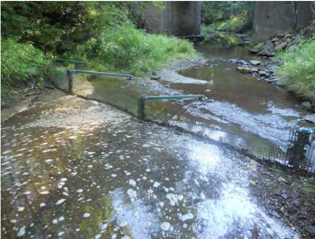
PICTURE SHOWING SANDBAR AT BOTH BARRIER
