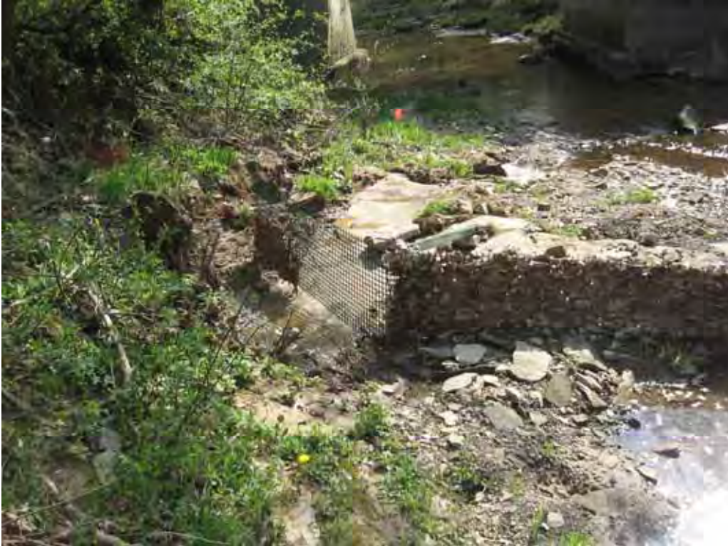
Picture showing north end of the bottom screen detached from stream bank.
