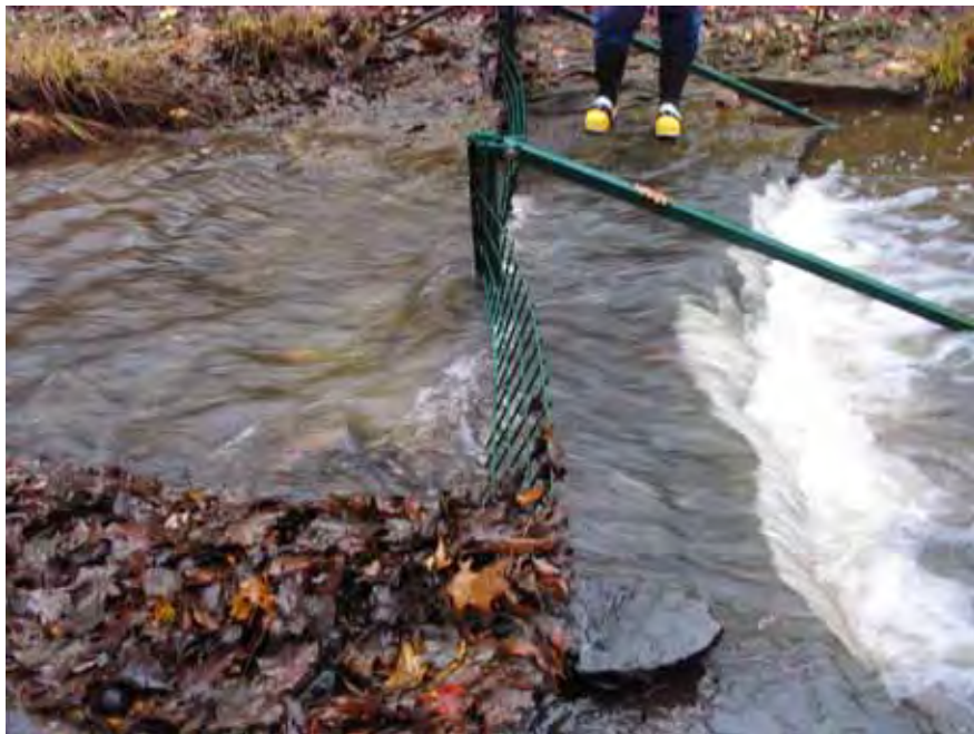
VIEW OF SLIGHT "BEND" NOTED IN THE UPSTREAM BARRIER.
