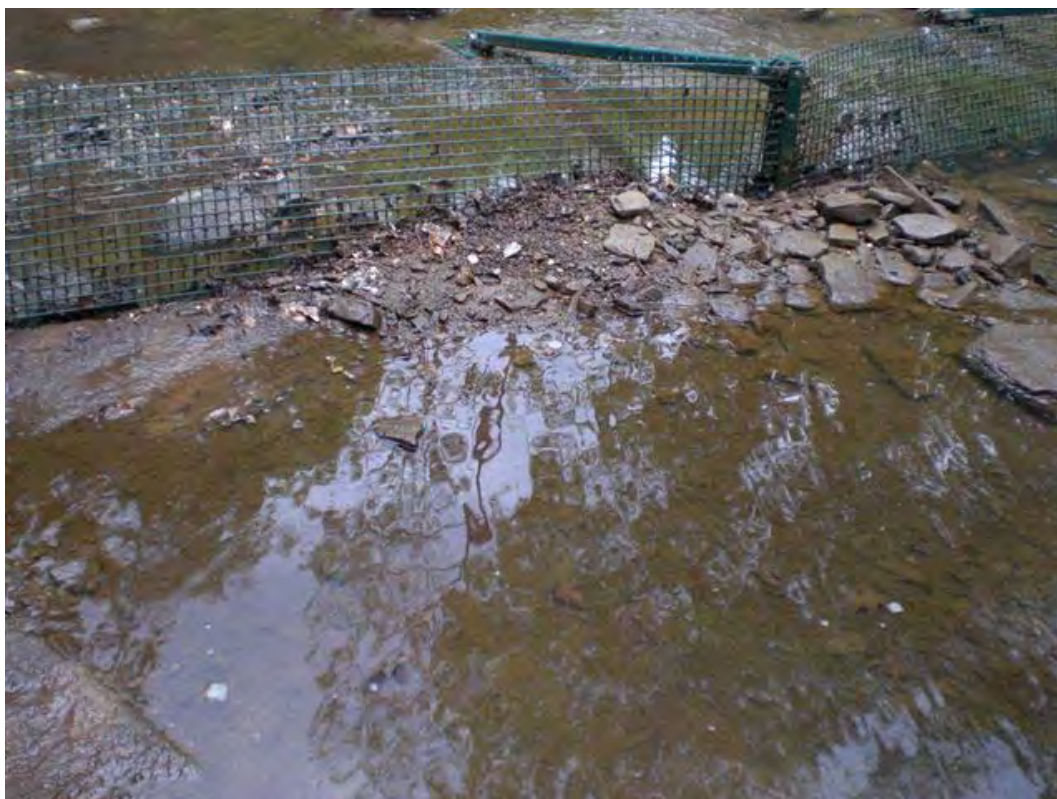
Photo 6: Downstream barrier, sand and gravel accumulation (27 May 2009)
