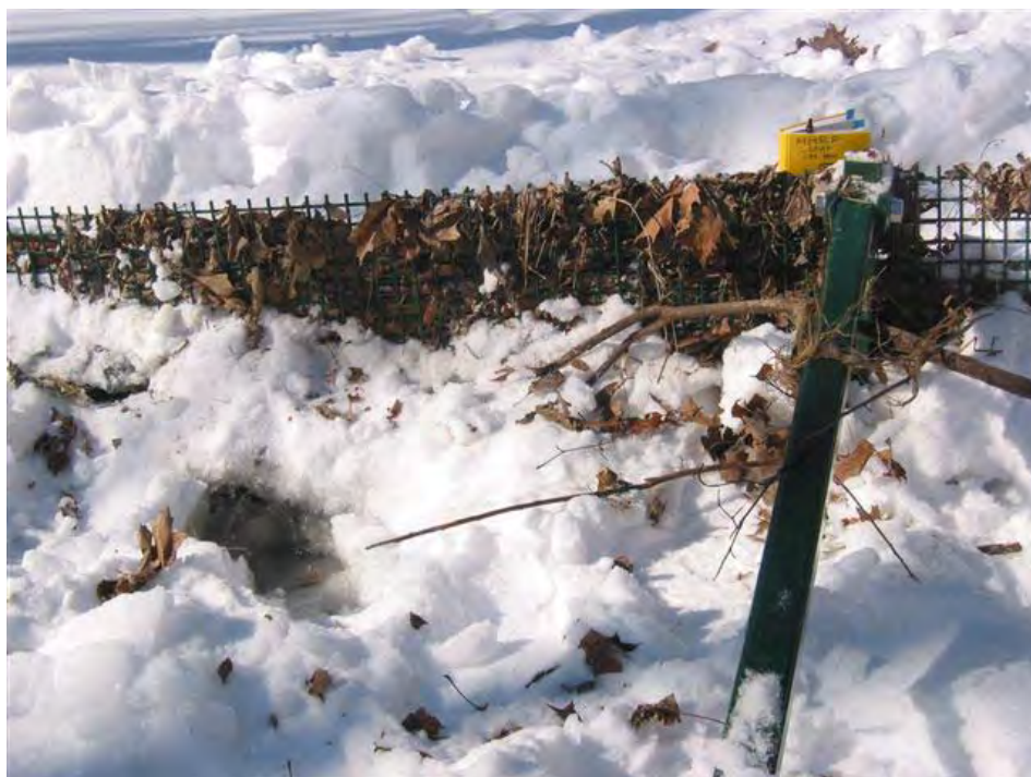
Photo 5: Post, back brace, and screen (12 December 2008)
