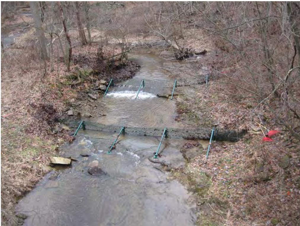
Overview of barriers following cleaning operations. Note: Remaining debris seen on screens is frozen to the screens.
