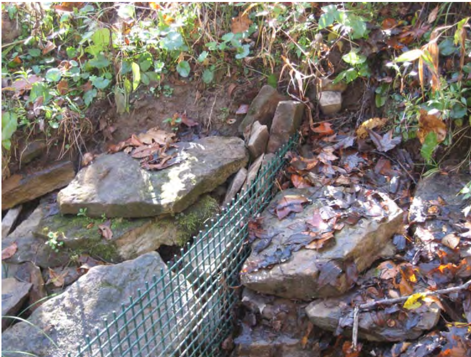
Washout area reinforced with rocks
