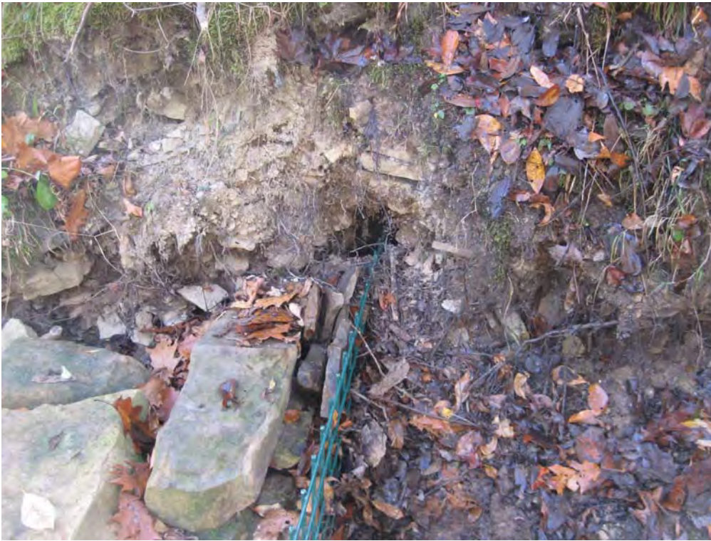
Washout area at barrier
