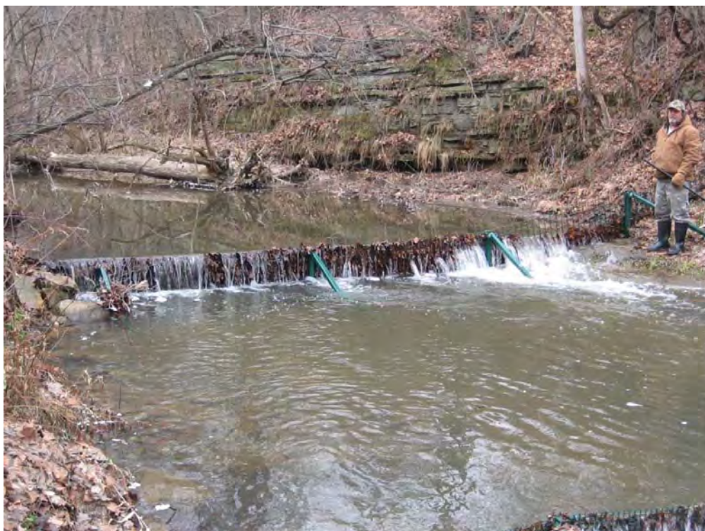
Photo 1: Upstream barrier loaded with leaves (12 December 2008)
