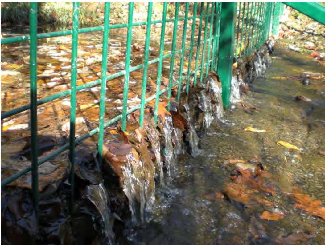
Photo 4: 7 – 8-inch deep leaves accumulated on the screen
