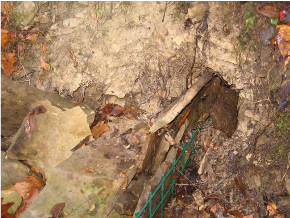
Washout area reinforced with rocks
