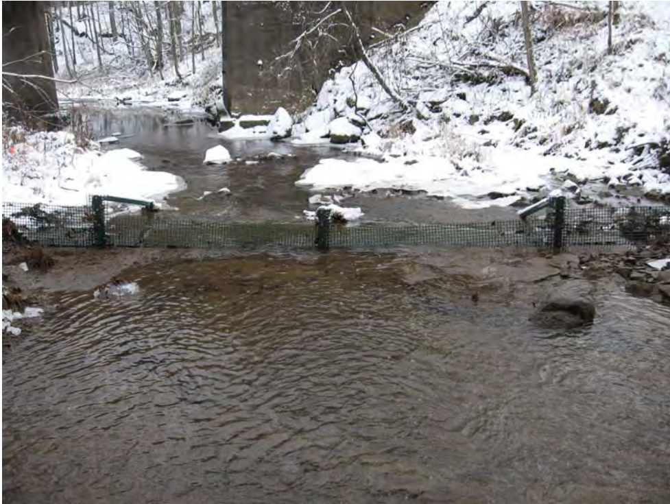
PICTURE SHOWING SILT BEGINNING TO ACCUMULATE ALONG DOWN STREAM SCREEN (LEFT).
