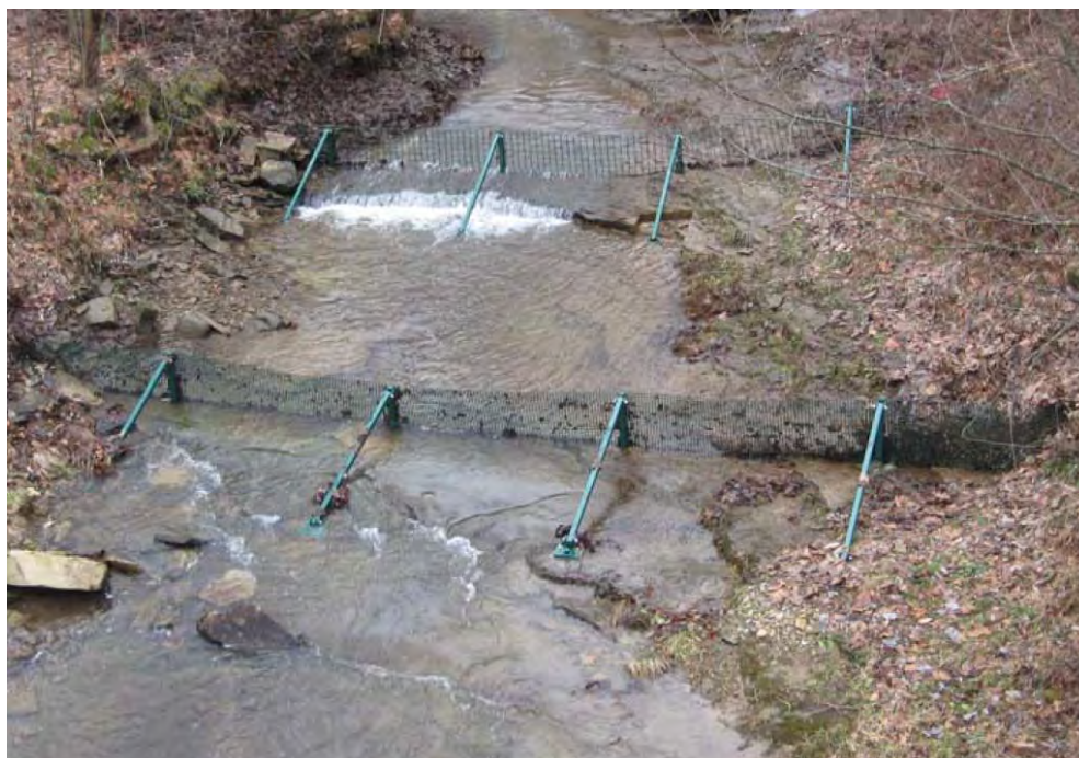
Photo 6: Barrier System after the 16 December 2008 O&M cleaning
