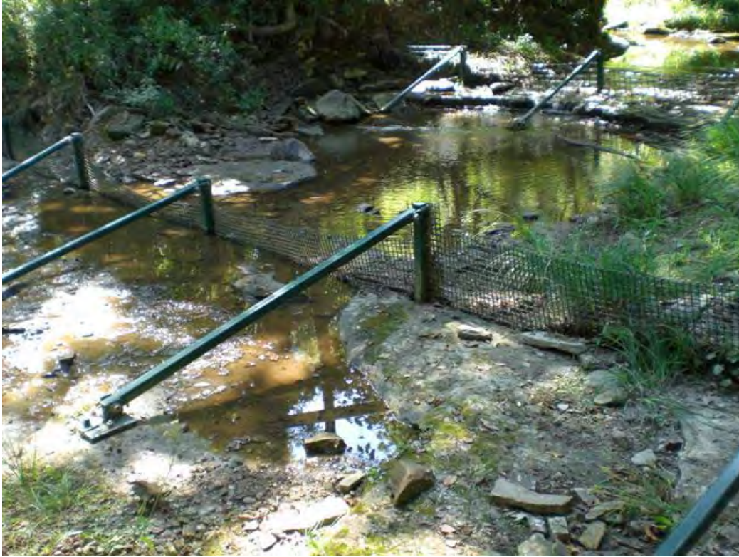
Photo 7: Downstream panels after height reduction (2 September 2009)
