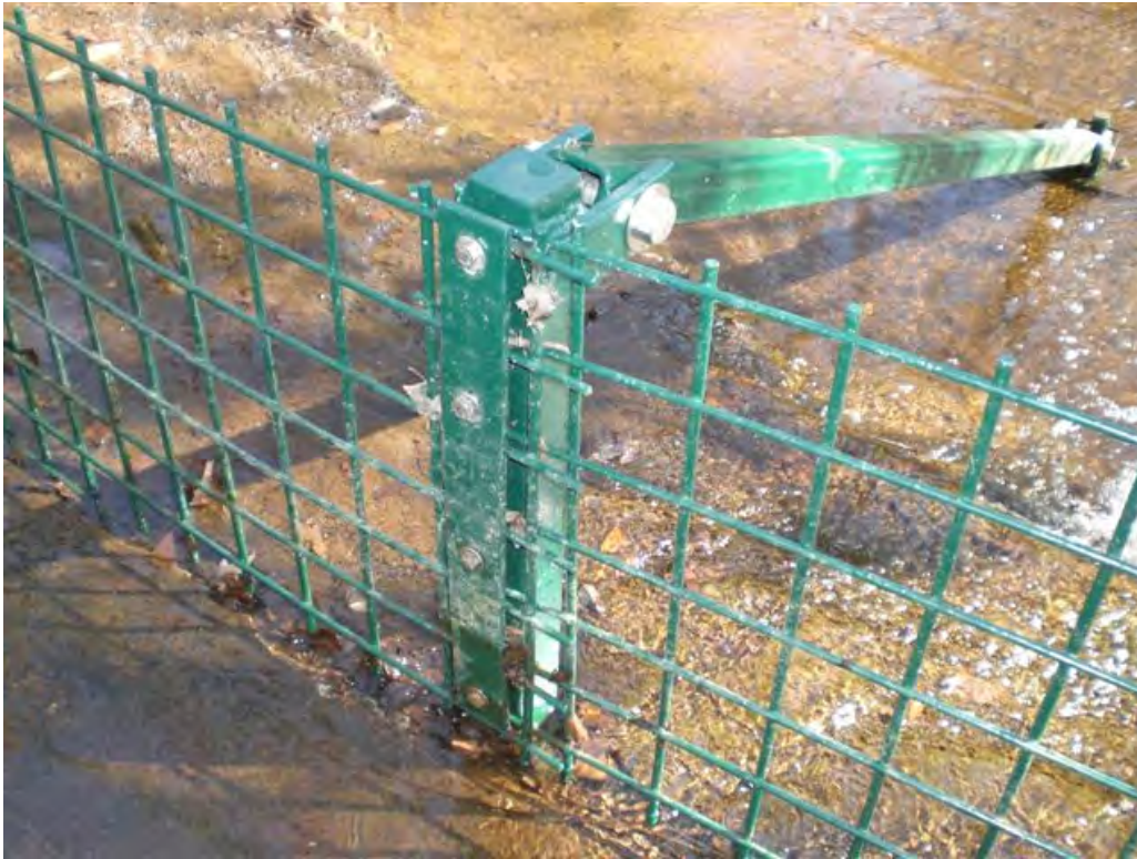
Photo 1: Upstream barrier post and back brace
