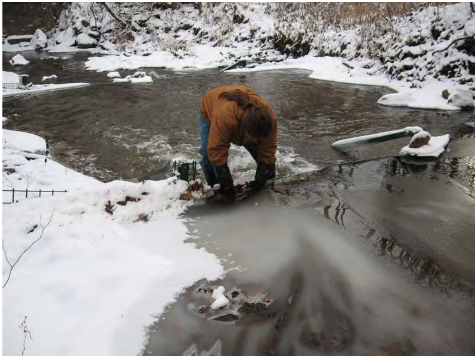
PICTURE SHOWING UXO TECHNICIAN REMOVING ACCUMULATED DEBRIS FROM SCREENS.
