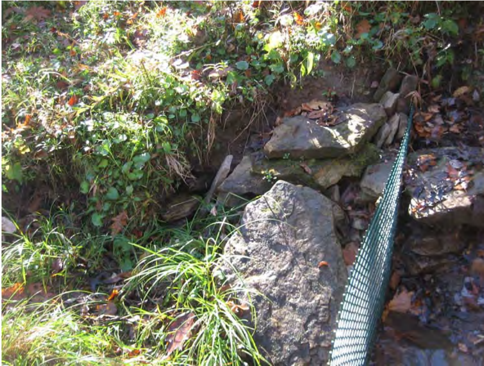
Washout area at barrier
