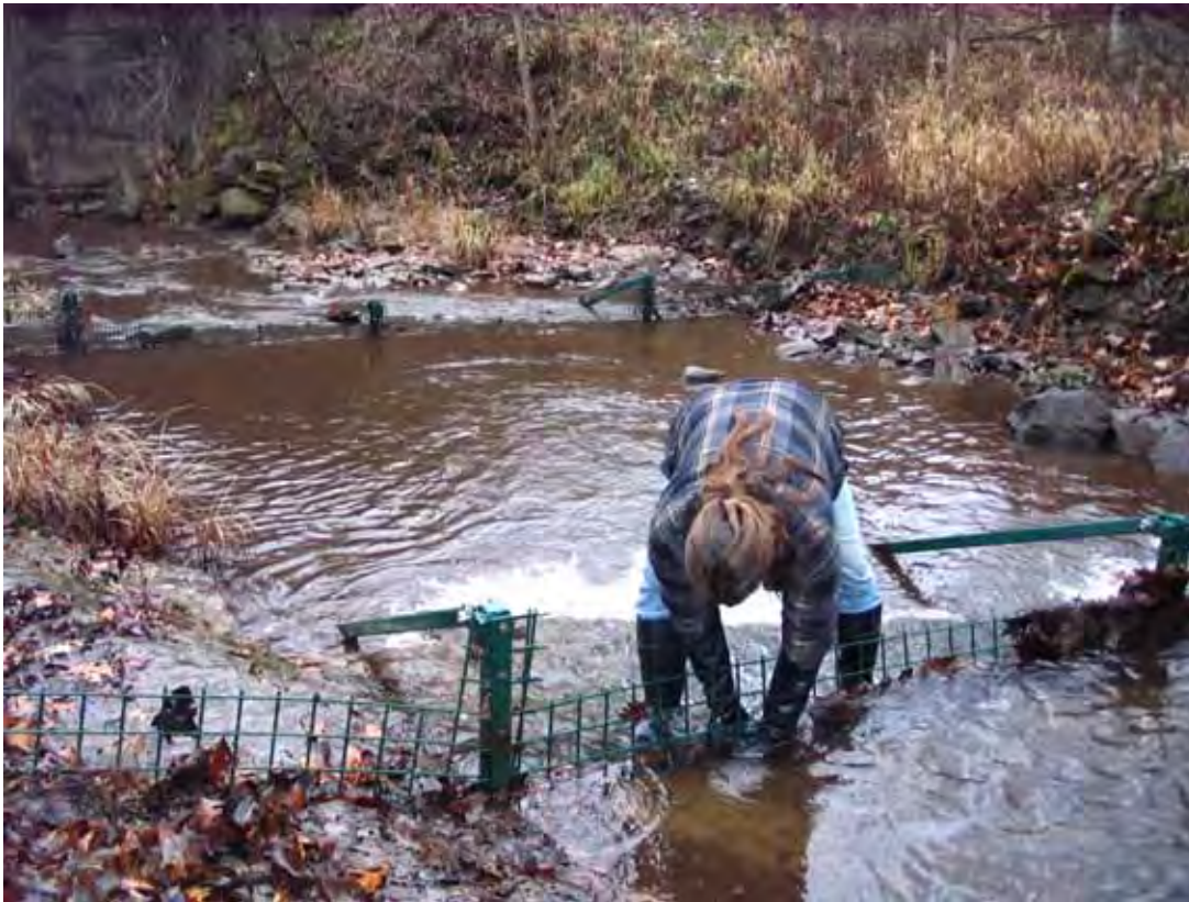
PICTURE SHOWING UXO TECHNICIAN REMOVING ACCUMULATED LEAVES FROM SCREEN.
