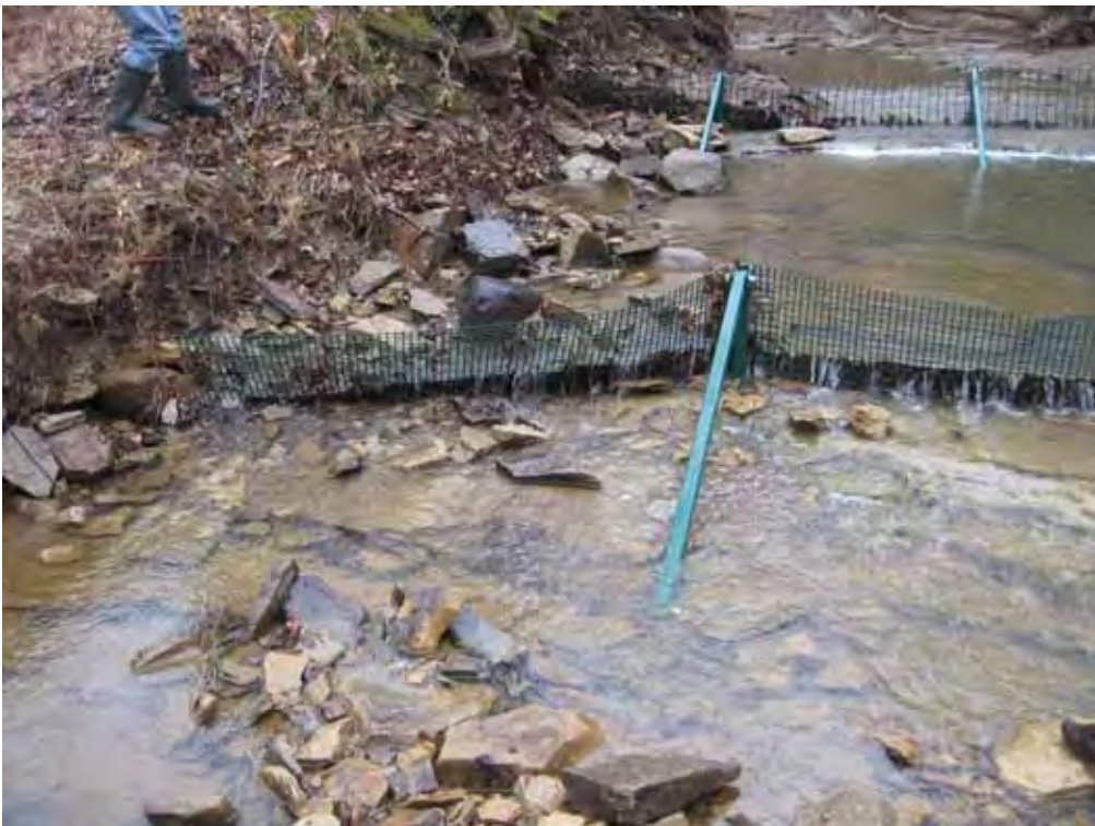
Pictures showing section of bottom screen detached from bank.
