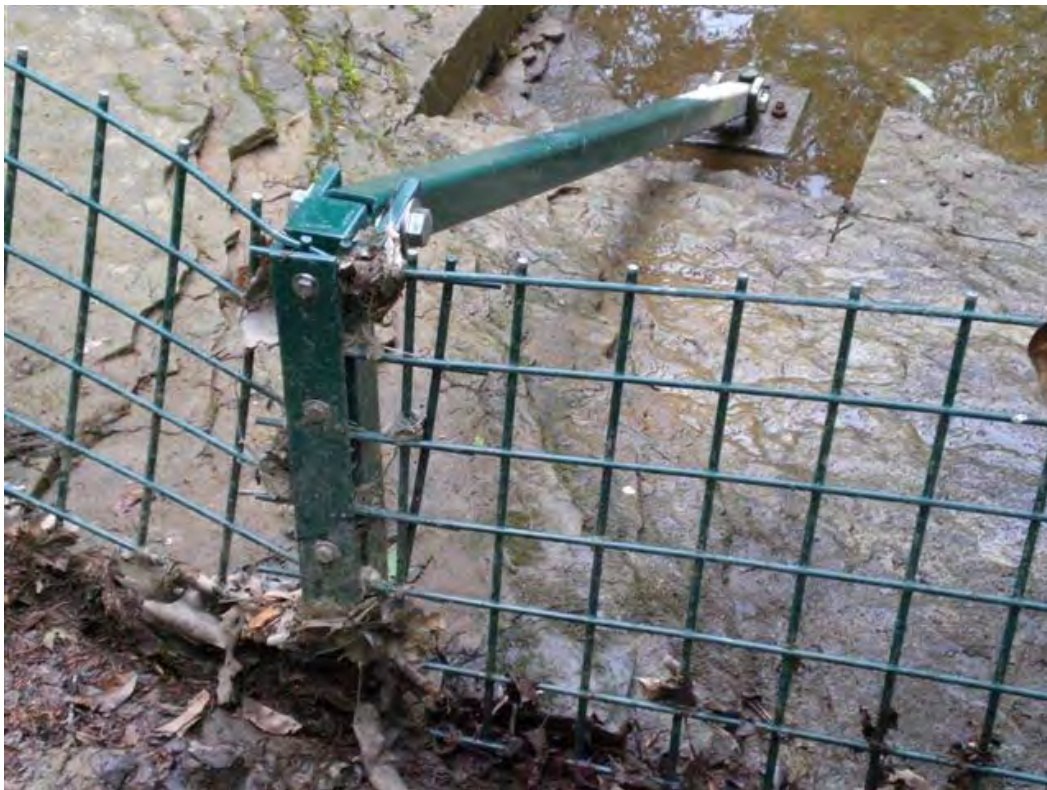
Photo 2: Upstream barrier, post and back brace (27 May 2009)
