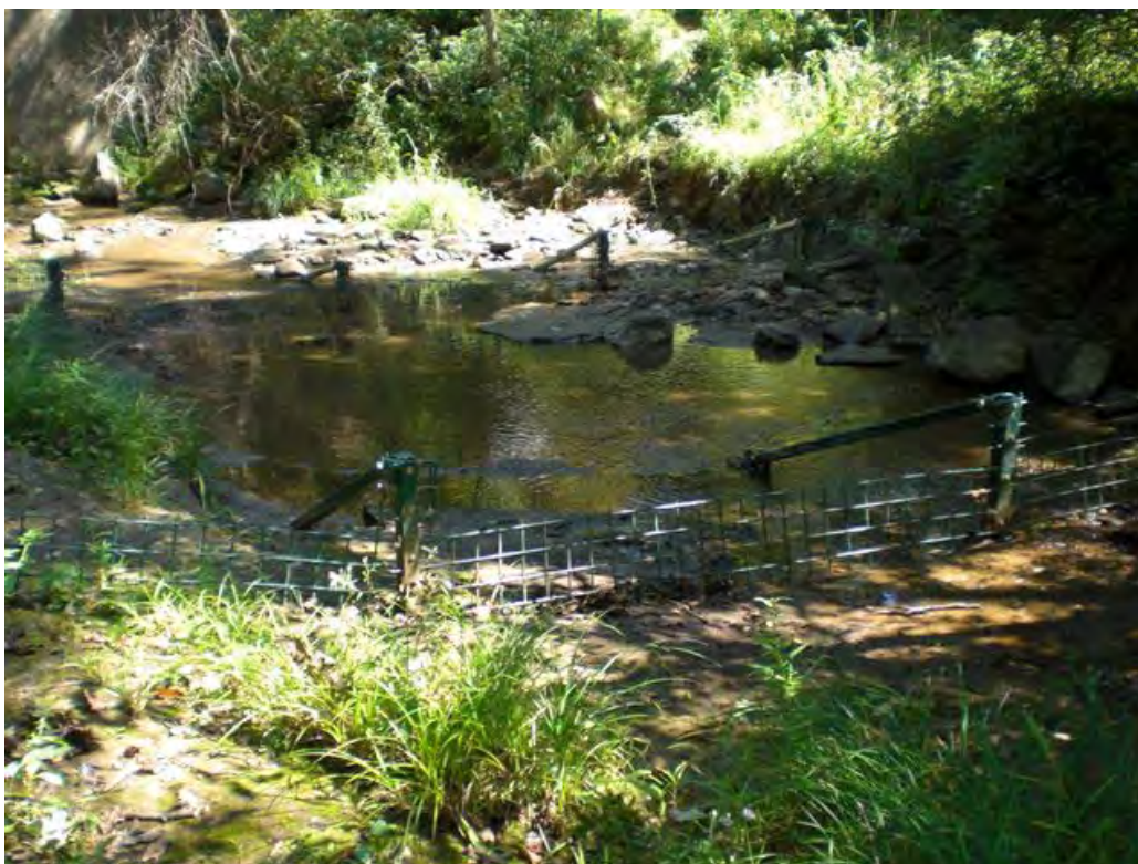
Photo 6: Upstream panels after height reduction (2 September 2009)
