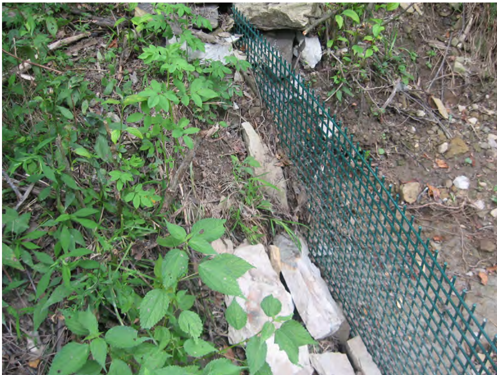
Washout area reinforced with rocks
