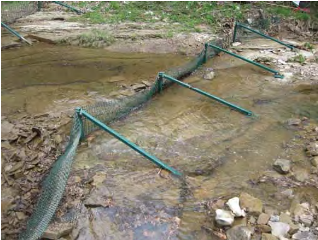
Picture showing south end of the bottom screen detached from stream bank.
