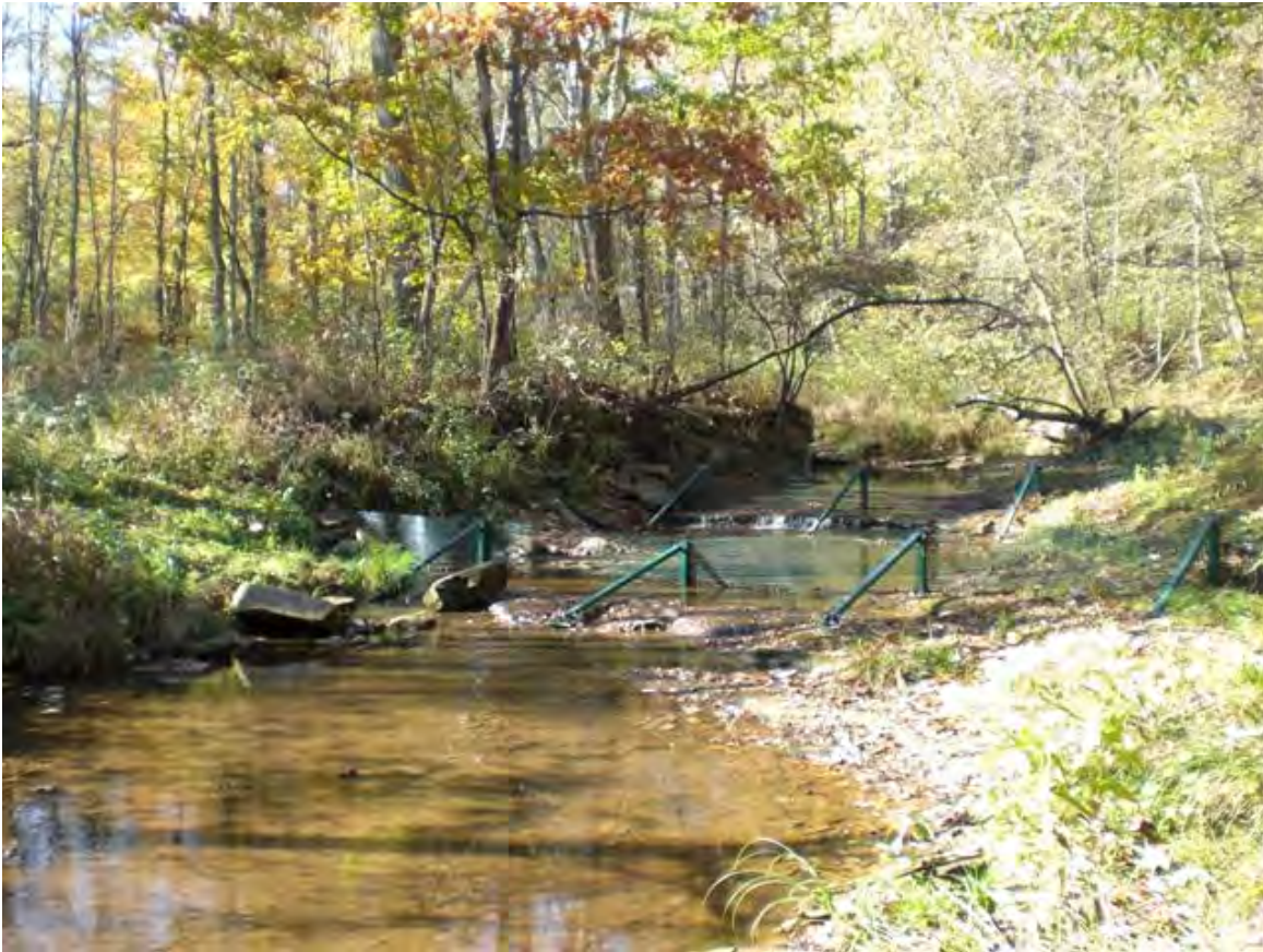
Photo 7: Barrier System, looking upstream
