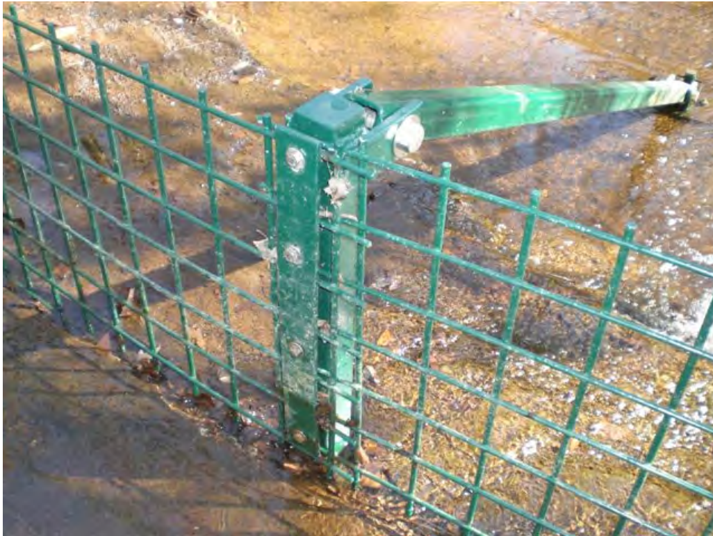
Photo 1: Upstream barrier post and back brace
