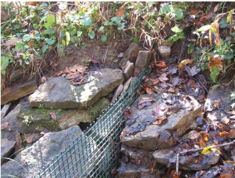
Washout area reinforced with rocks
