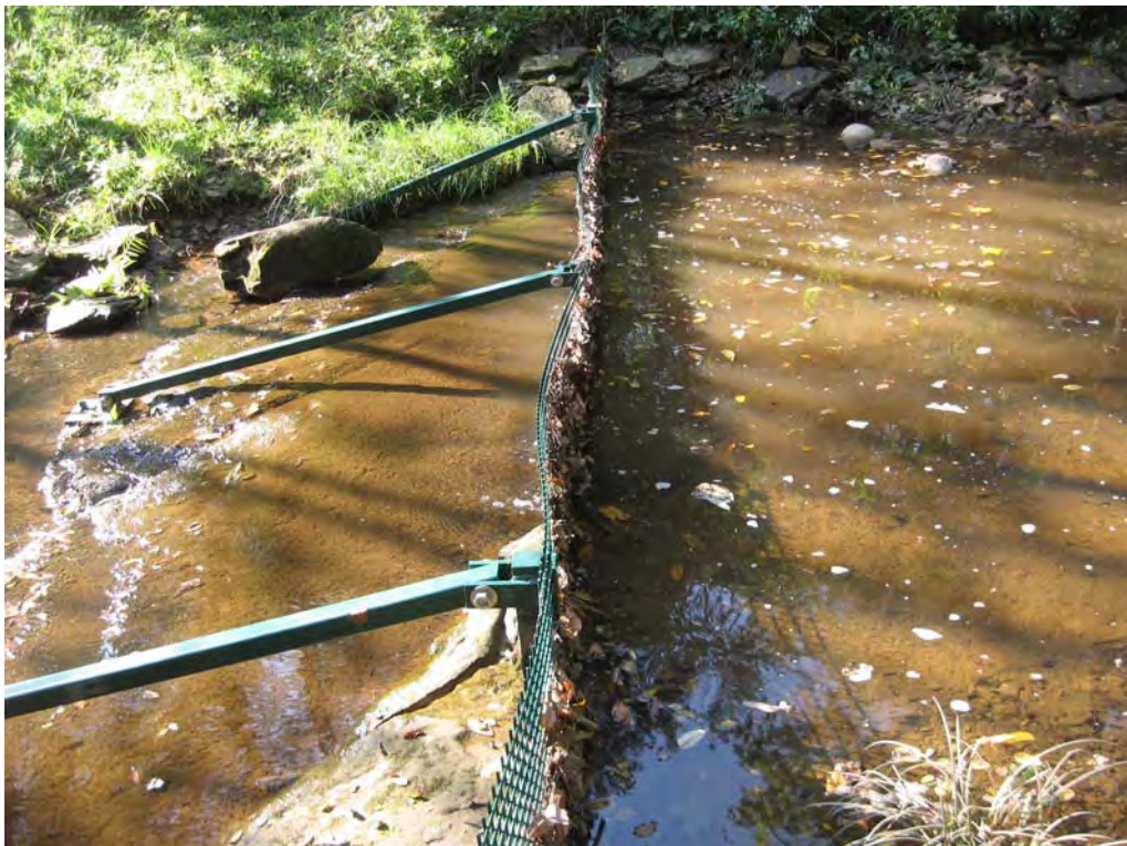
Bowing of barrier
