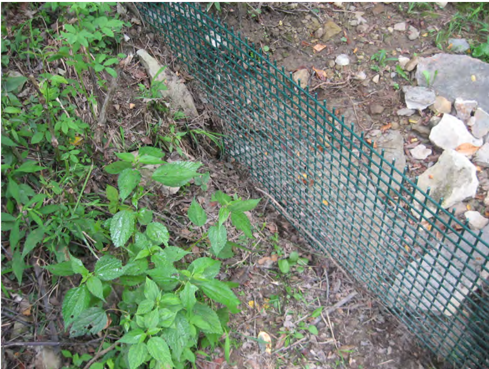
Washout area at second barrier
