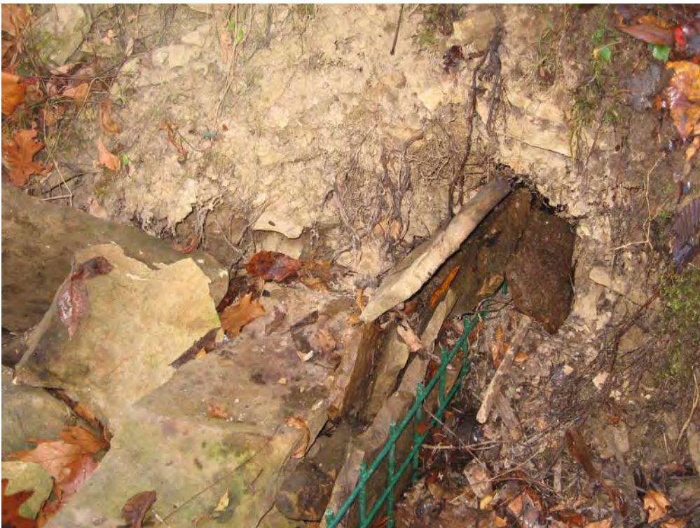
Washout area reinforced with rocks
