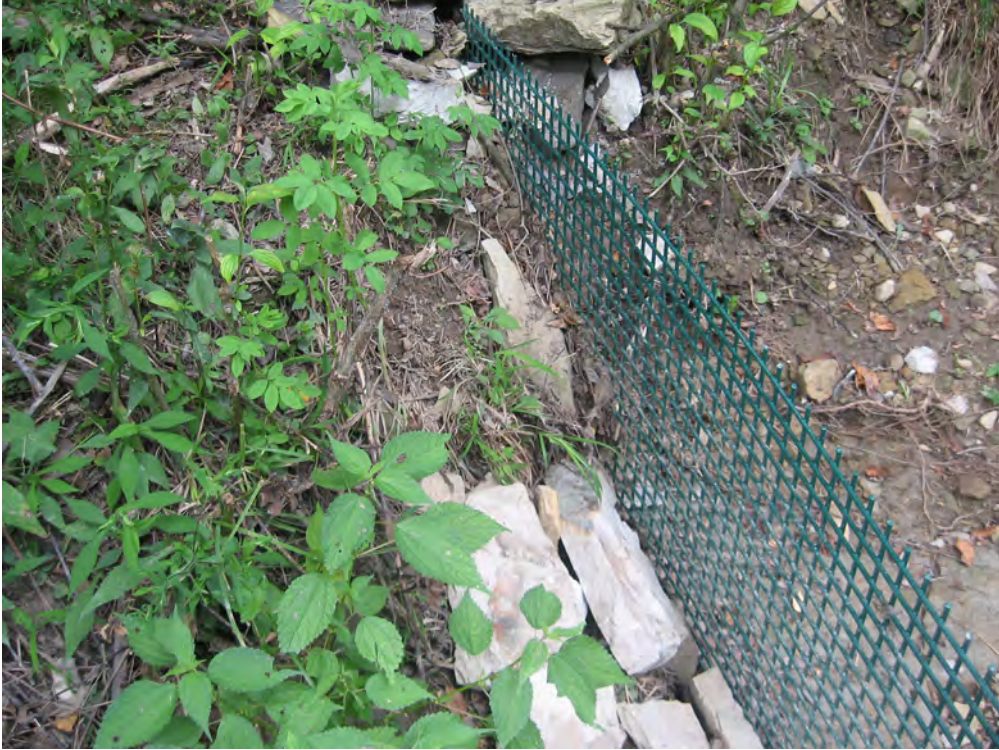
Washout area reinforced with rocks
