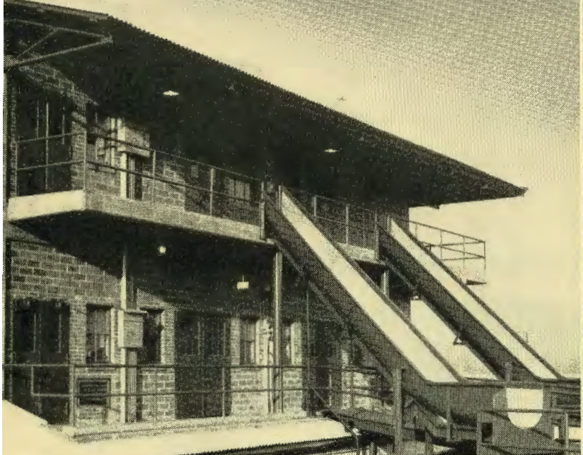
Safety chutes have been installed in all buildings where explosives are handled. These chutes are designed to enable employees to get out of the buildings or danger zones as quickly as possible. Installed near these chutes are "deluge rings," which flood with water rooms in which explosives are being used.
