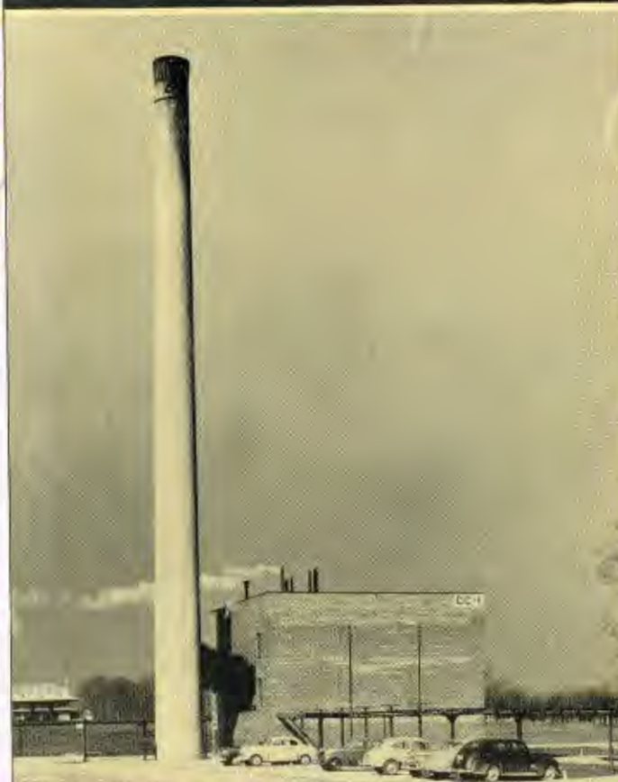
Below is shown a typical Power Unit. Note safety rods at top of smoke stack.
