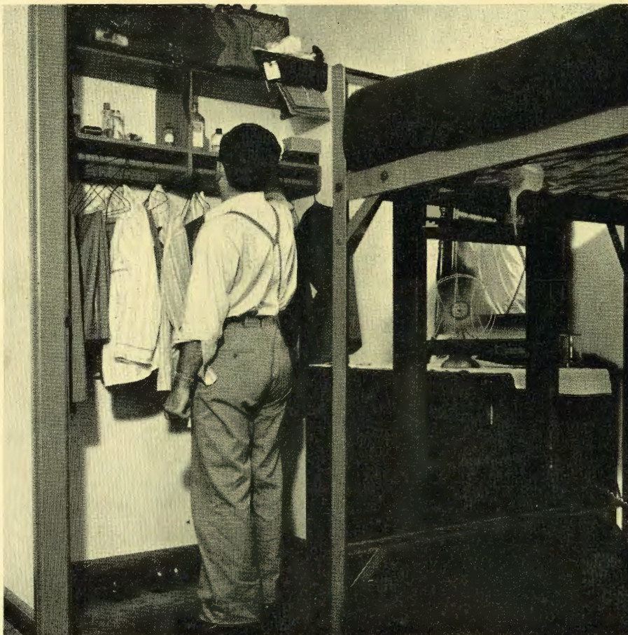
Interior of one of the School's dormitory rooms is shown above. Two men are stationed in each of the rooms, equipped with double-decker beds, writing desks and wardrobes.
