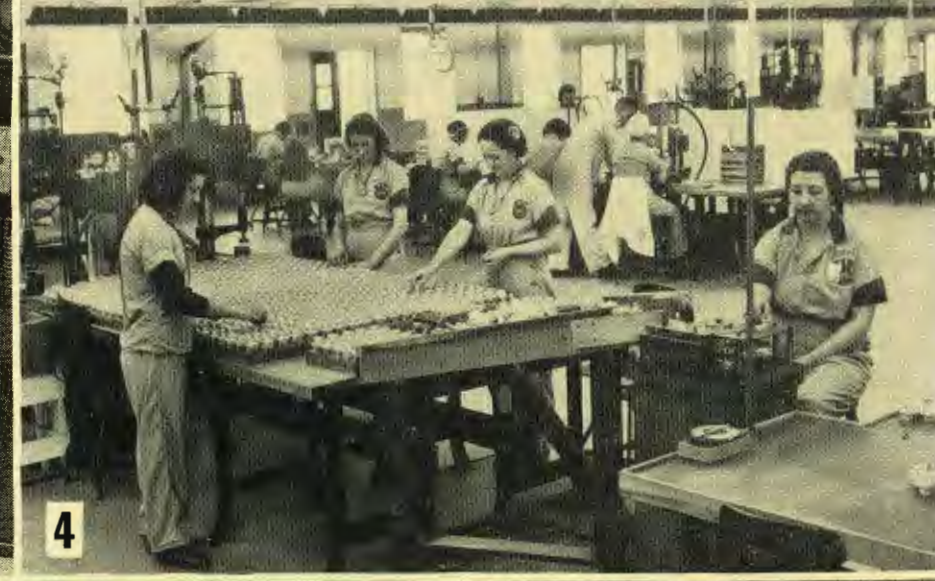
Fuze bodies are stamped for identification and loaded with plunger bodies. Shown, left to right, are Yolando Dinardo, Rose Chupak, Geraldine Zimmerman, and Isabel Murphy.
