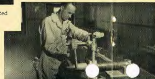
A fuze is attached and tensioned.
