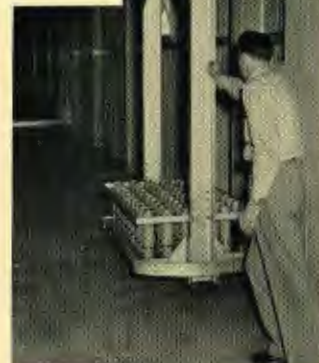
A long trip through a ramp to the pouring boys.
