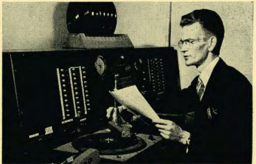
Pictured above is Joe Mulvey reading an announcement over the public address system from the central control room. In the foreground can be seen the "recording arm". The buttons on the panel are the switches which control the outlets.
