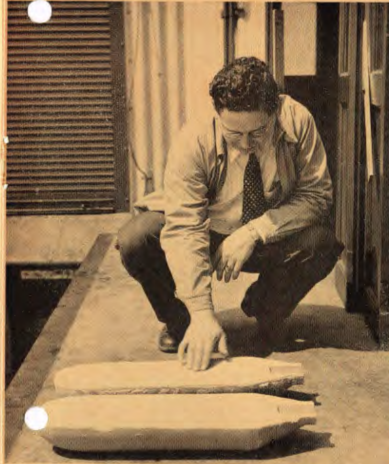
Inspector Edward J. VanArnhem is checking a split bomb casting for cavitations.
