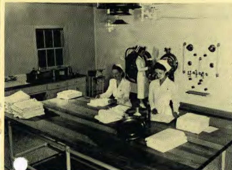
... Central Supply Room
