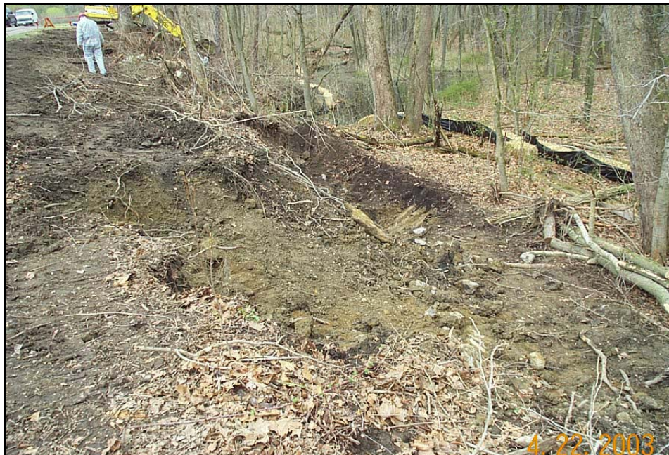
Photograph 3-1. Debris Removal Activities Near Grid #4 and Grid #5, April 2003
