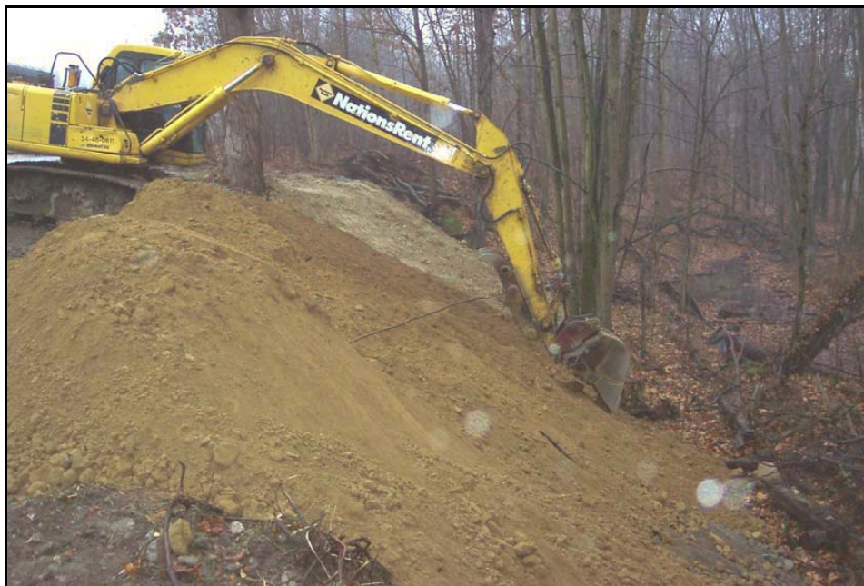
Photograph 3-2. Installation of Two-foot Soil Backfill Cover During Restoration Activities, November 2003
