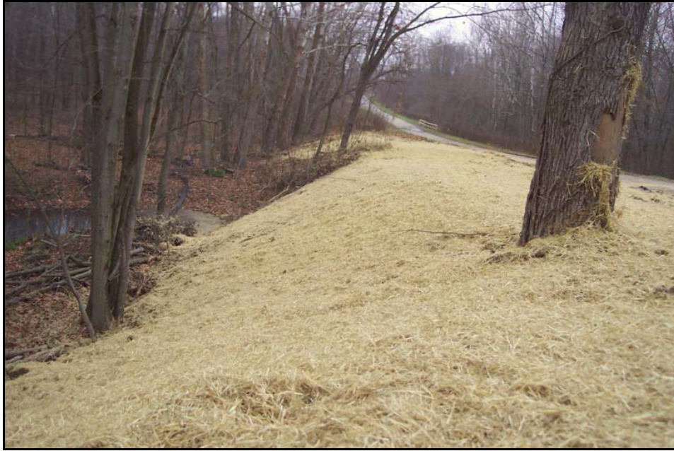
Photograph 3-3. Site Conditions at the Completion of Site Restoration Activities, November 2003
