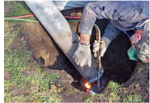
Cutting off the casing.
