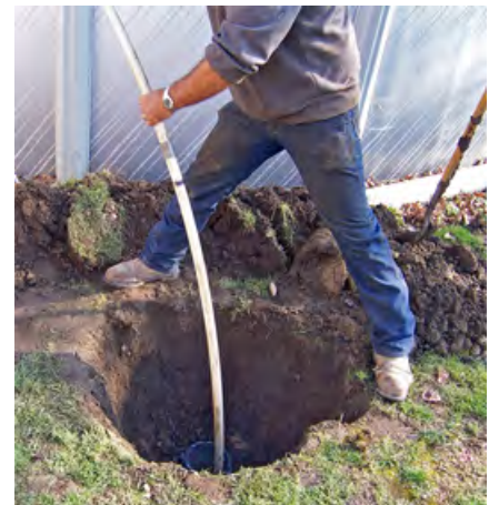
Pressure grouting – early stage.
