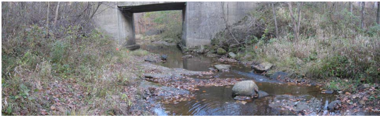
Photograph 3: Barrier system site
