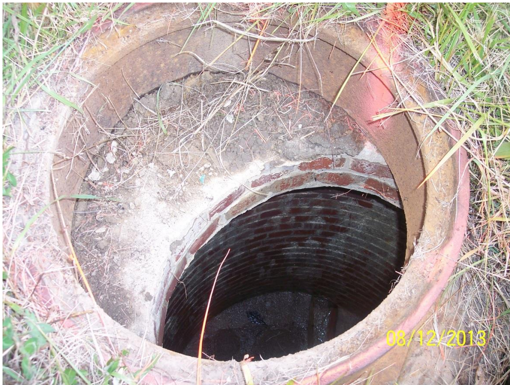
View is looking into the manhole. Note orange line on manhole rim aligns with incoming pipe visible in the bottom of the manhole.
