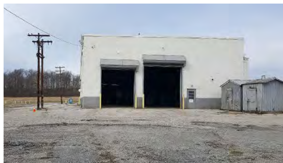
Photograph 1: Outside of Building 1034. View is from the back of the building facing west. The hydraulic lift is just inside the left roll-up door.
