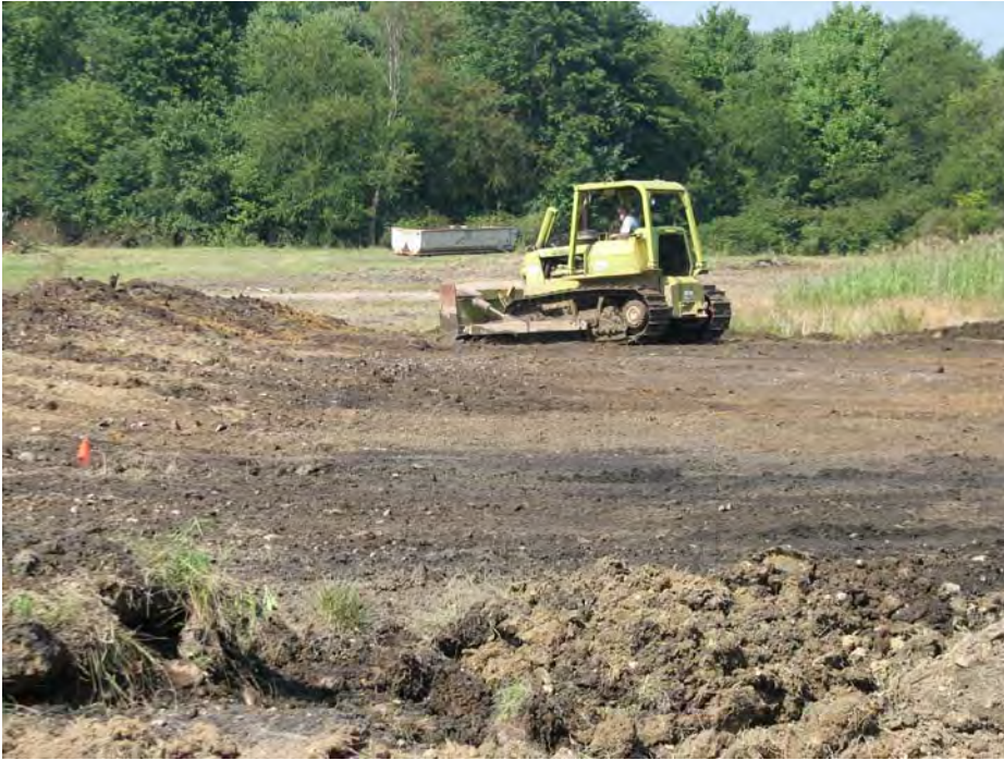
DLA Rt. 80 Tank Farm Site. Building berms with dozer.
