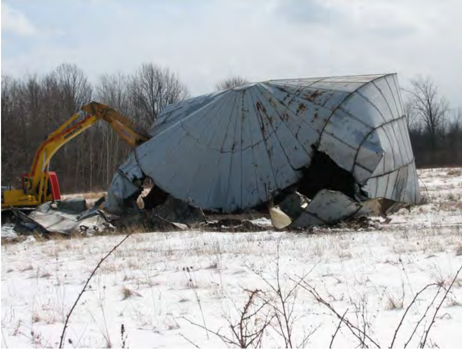
DLA Rt. 80 Tank Farm Site. AST being demolished with Excavator/shear.
