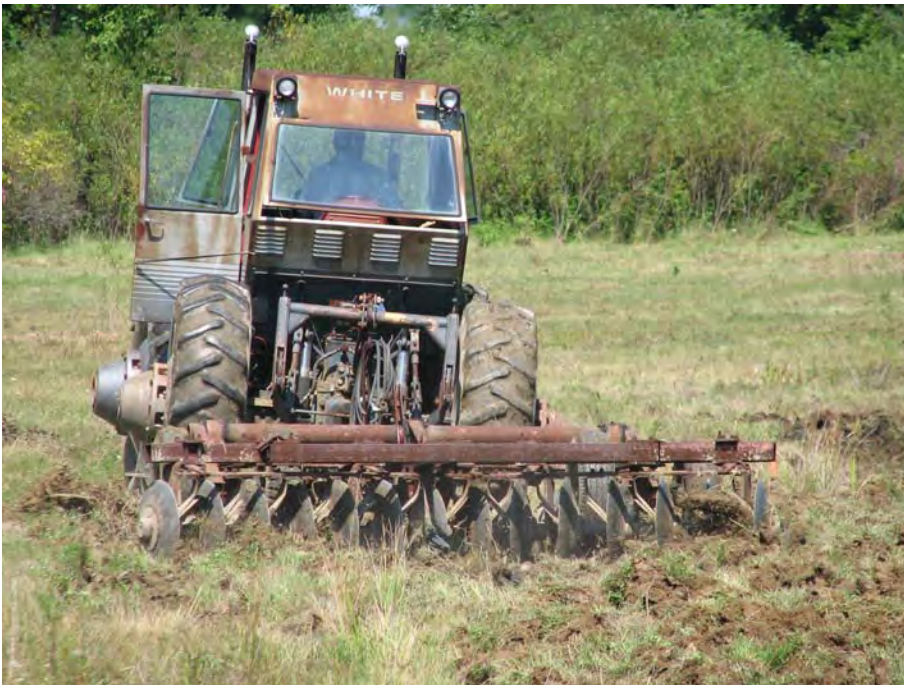
DLA Rt. 80 Tank Farm Site. Disking site prior to regrading.
