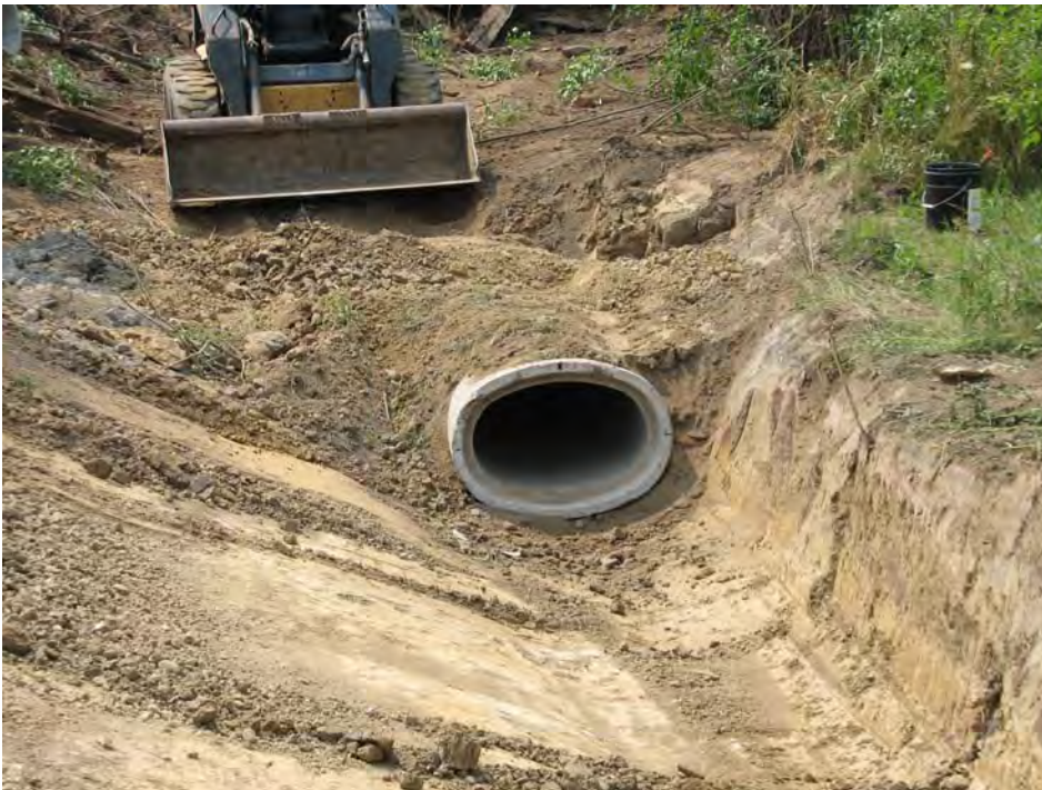
DLA East Ore Yard Site. Installing 24-inch elliptical concrete pipe.
