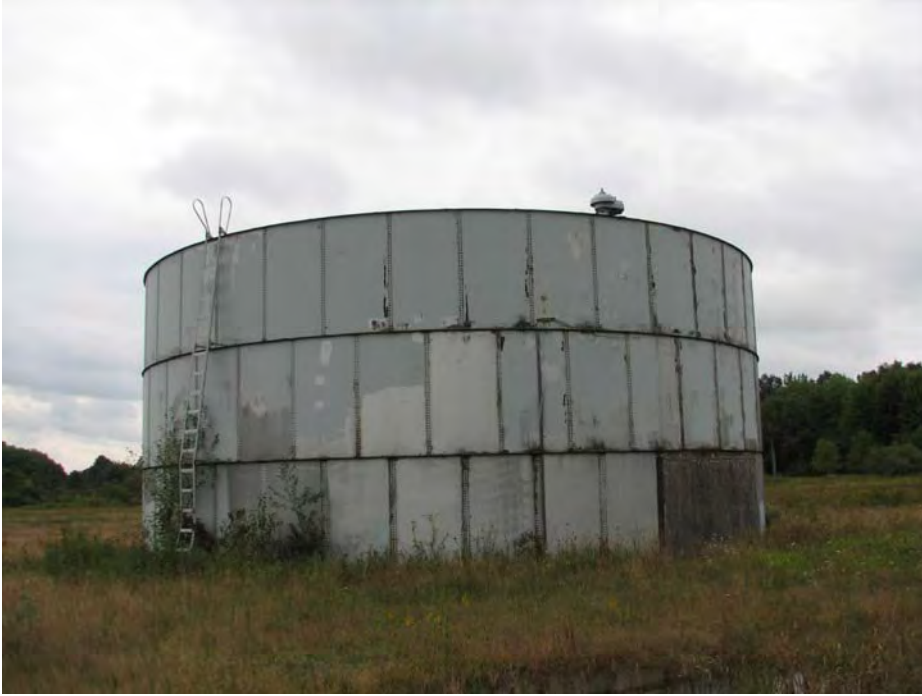
DLA Rt. 80 Tank Farm Site. Above-ground storage tank prior to demolition.
