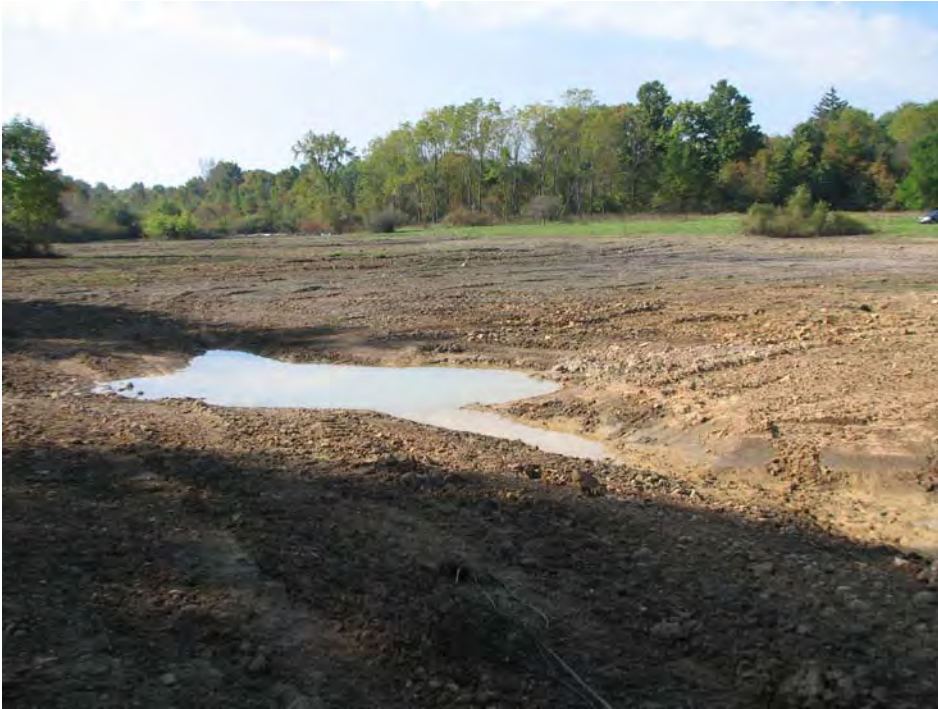
DLA Rt. 80 Tank Farm Site. Re-graded site with constructed hollow area.
