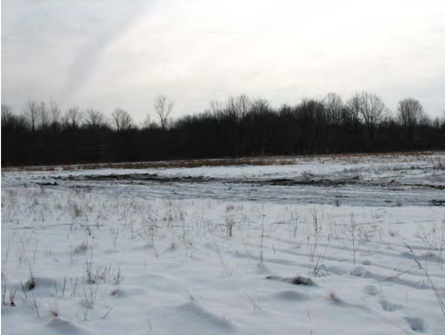
DLA Rt. 80 Tank Farm Site. Immediately after AST demolition and site cleaning.
