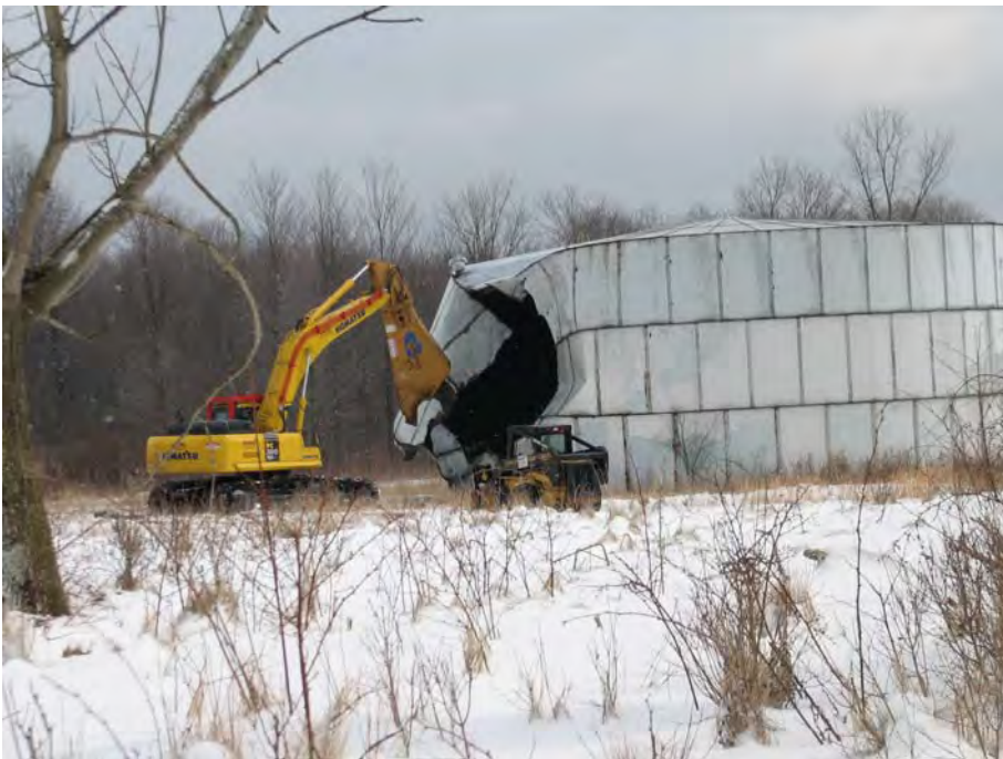
DAL Rt. 80 Tank Farm Site. AST being demolished with Excavator/shear.
