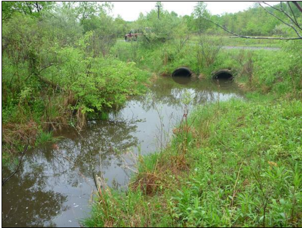
Photograph H-1. Active Area Channel at Load Line 12 (looking northeast from the old railroad bed east of the Former Settling Pond on May 18, 2010)
