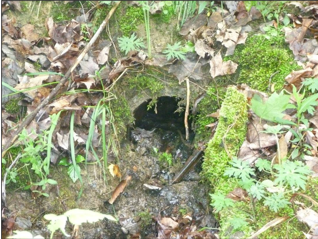
Photograph H-4. Close-up of Outlet at Load Line 11 (May 19, 2010)
