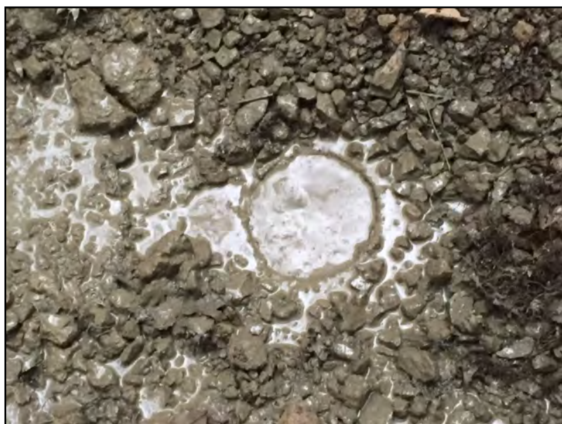
Well 37 following grouting
