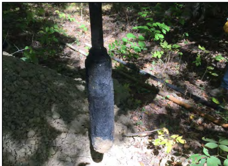
Pump and piping removed from Well 100.
