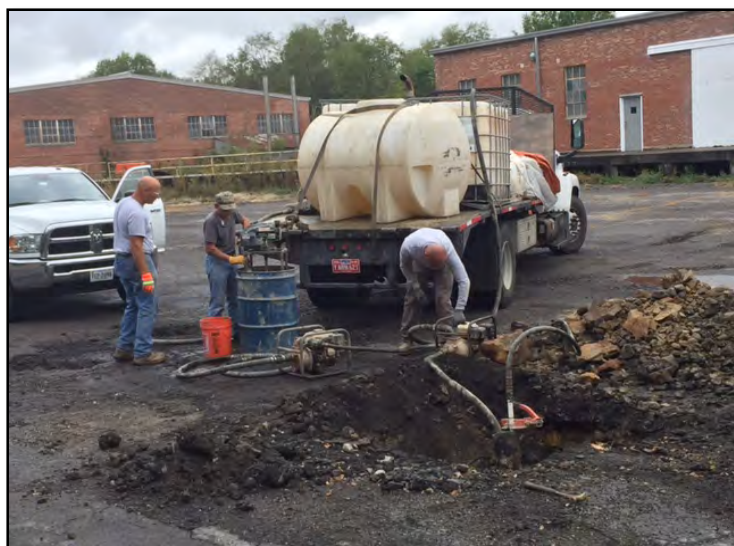
Well 31 during grouting.
