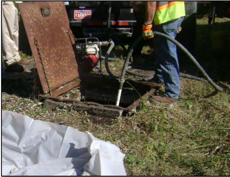
Well 7 during grouting.
