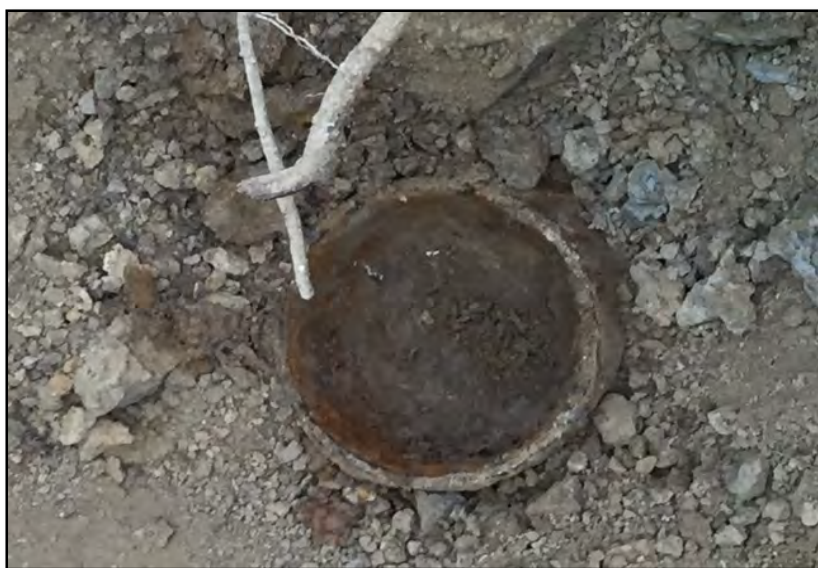
Exposed top of casing at Well 32 with historical grout shown.
