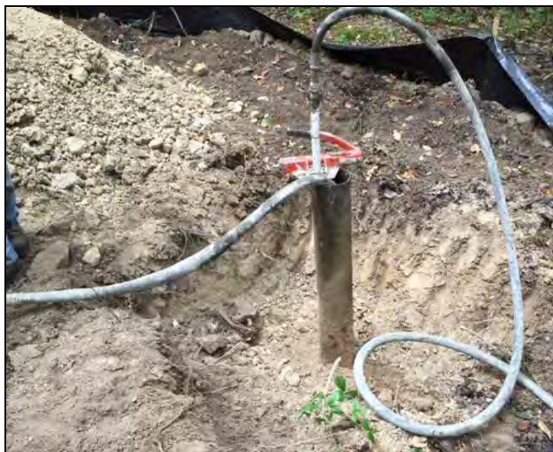
Well 54 during grouting.
