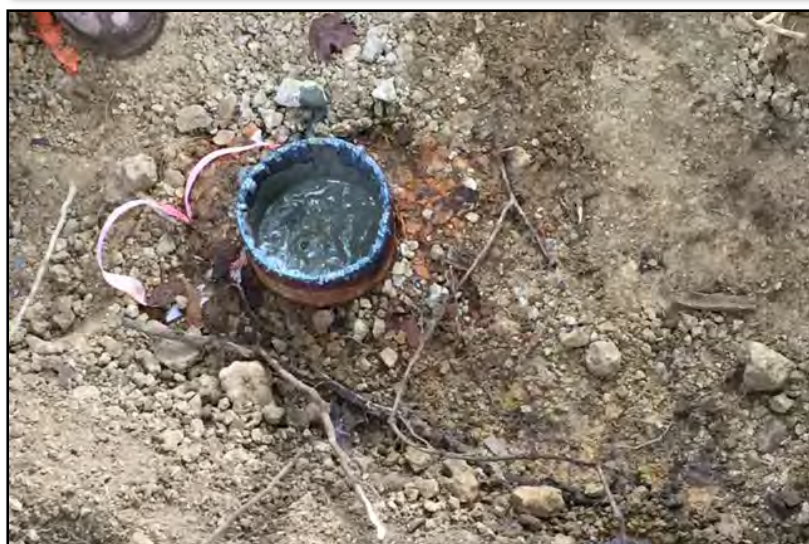
Well 56 at completion of grouting.
