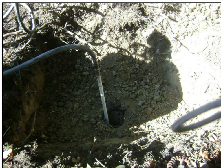
Well 39 during grouting.
