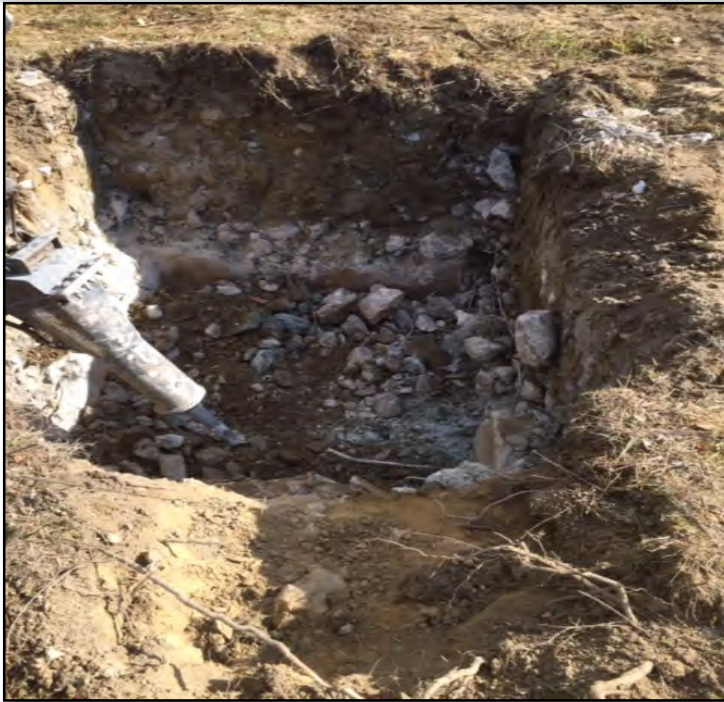
Well 7 during concrete vault removal.
