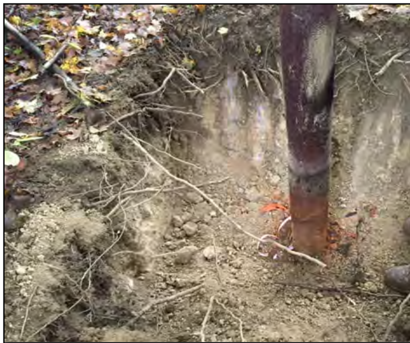
Well 56 with casing exposed.
