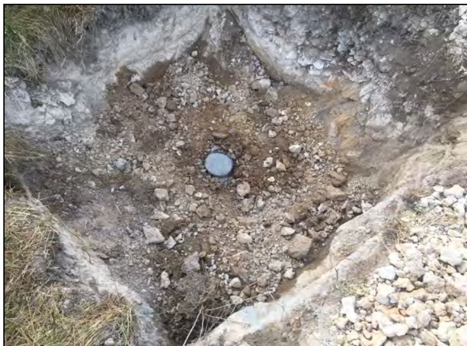
Well 50 at completion of grouting.
