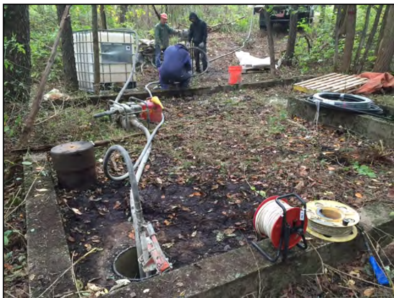
Well 49 during grouting.
