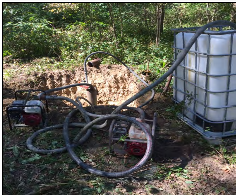
Well 14 during grouting.
