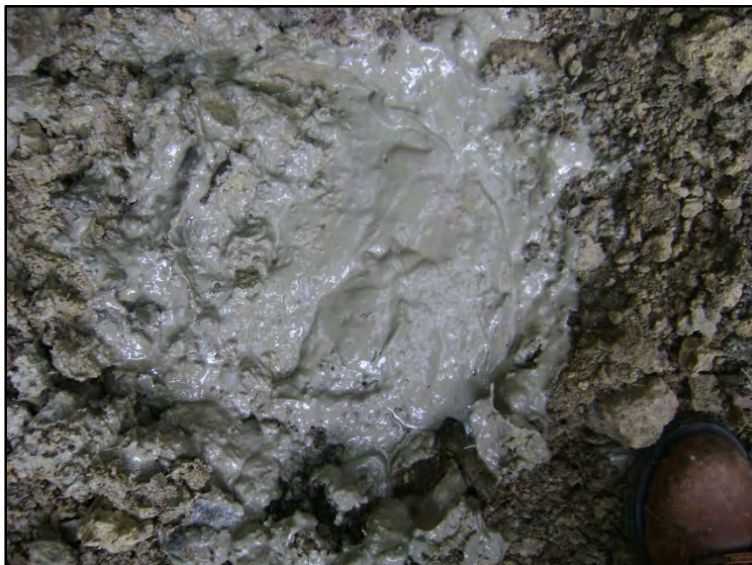
Well 3 following grouting.
