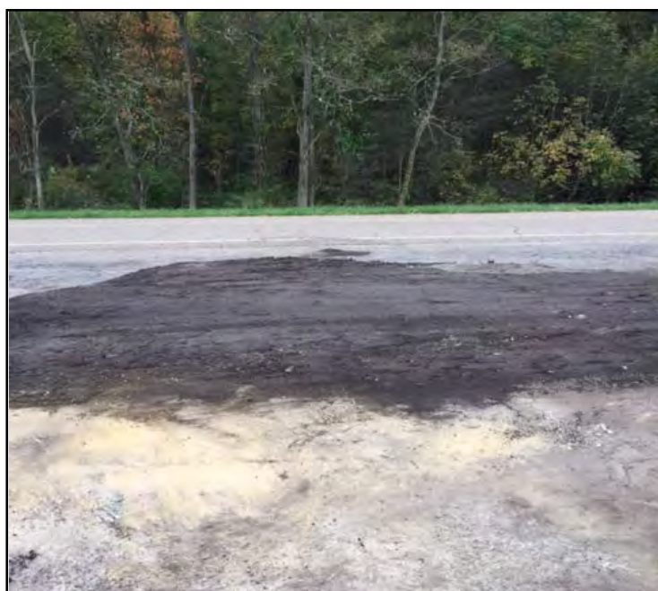
Well 31 following backfill and surface restoration.
