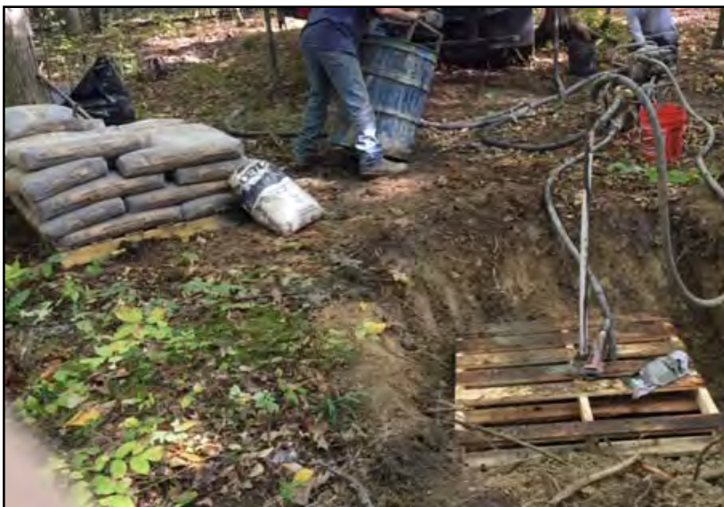
Well 62 during grouting.
