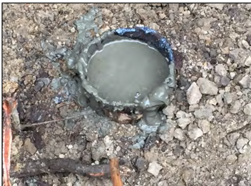
Well 66 at completion of grouting.
