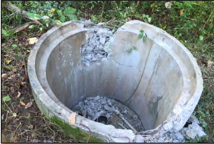
Well 95 during concrete removal.
