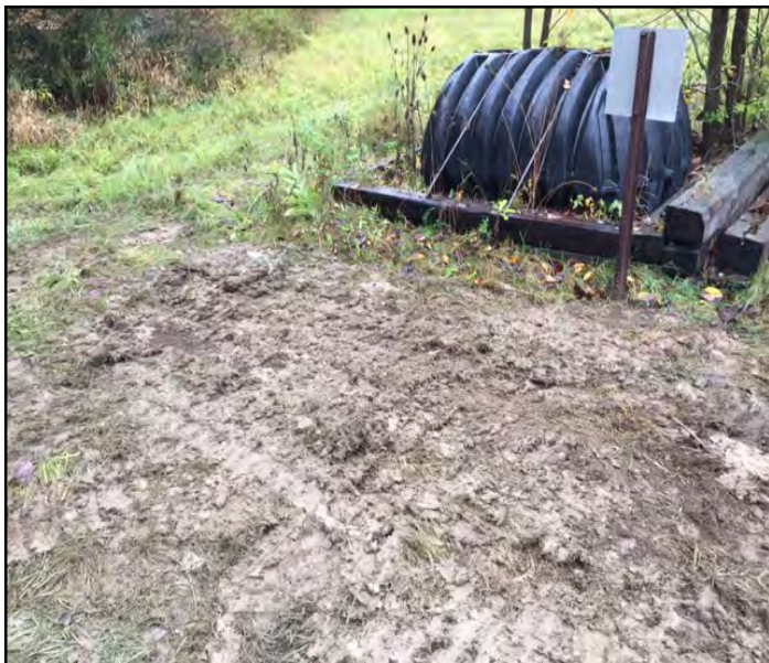
Well 98 following backfill.
