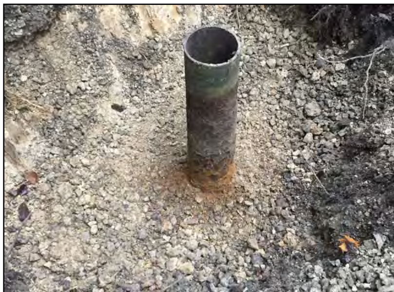
Well 37 with casing exposed.
