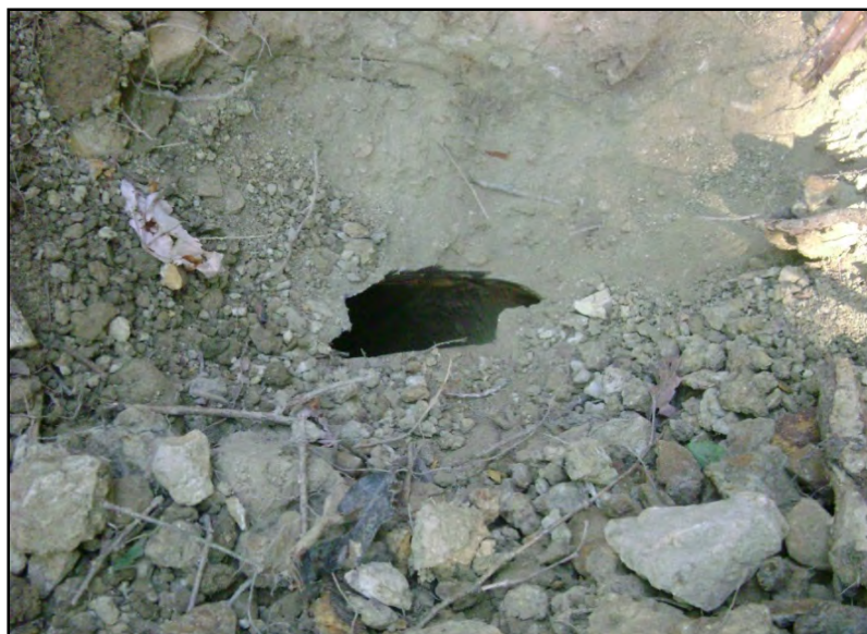
Well 38 with broken buried casing exposed.
