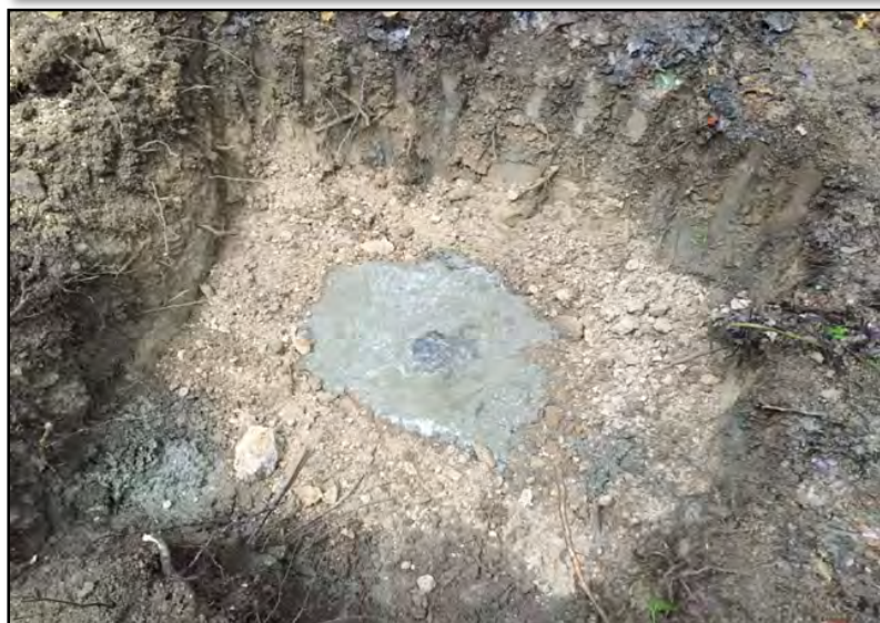
Well 54 at completion of grouting.
