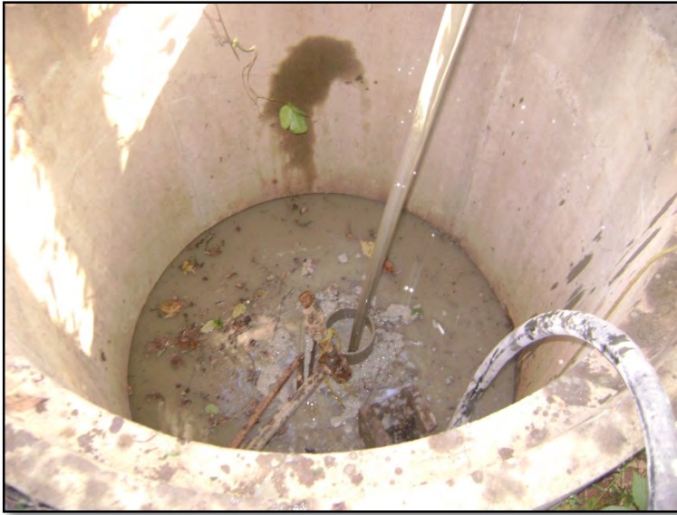
Well 95 during grouting.
