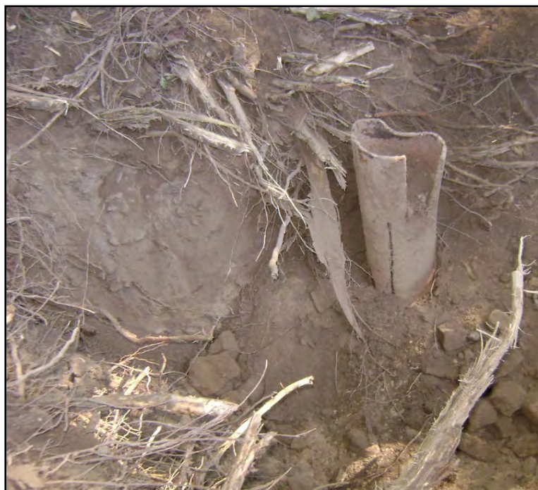
Well 39 with casing exposed.
