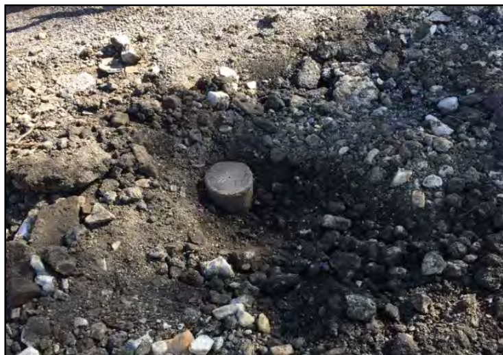
Well 31 following casing exposure
