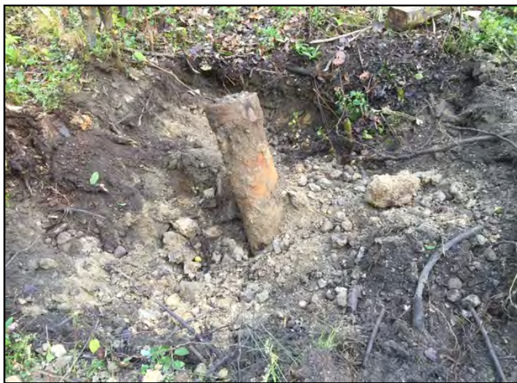
Well 5 with casing exposed.
