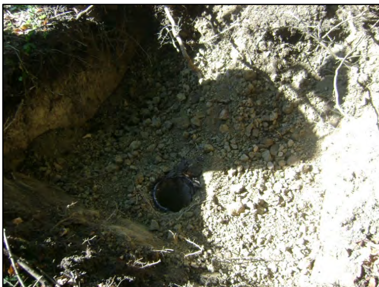
Well 3 following casing being cut and prior to abandonment.
