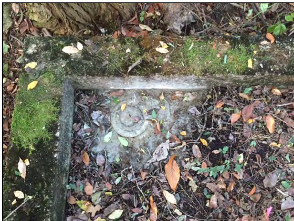
Well 49A at completion of grouting.
