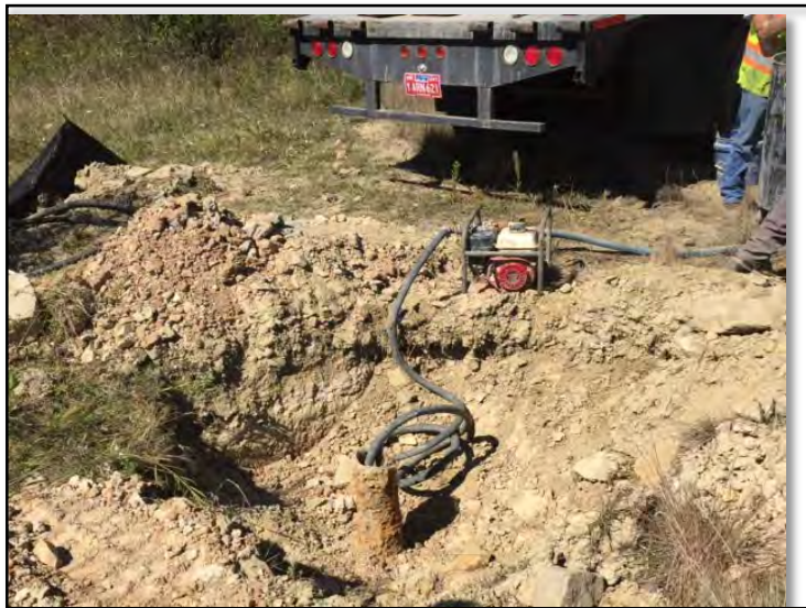
Well 51 during grouting.
