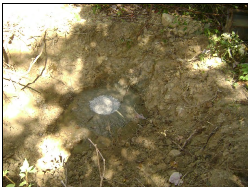
Well 38 following grouting.
