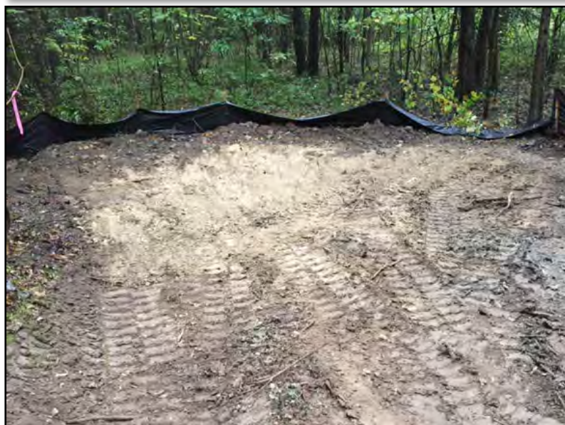
Well 54 following backfill.
