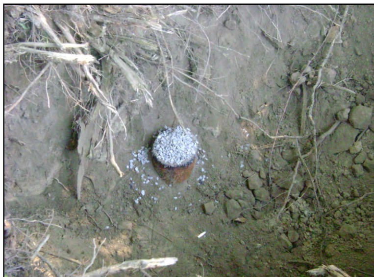
Well 39 following completion of grouting.
