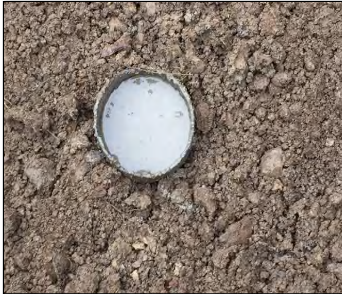
Well 98 following grouting.
