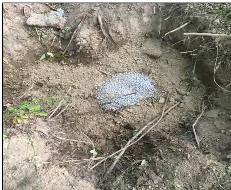
Well 100 following grouting.
