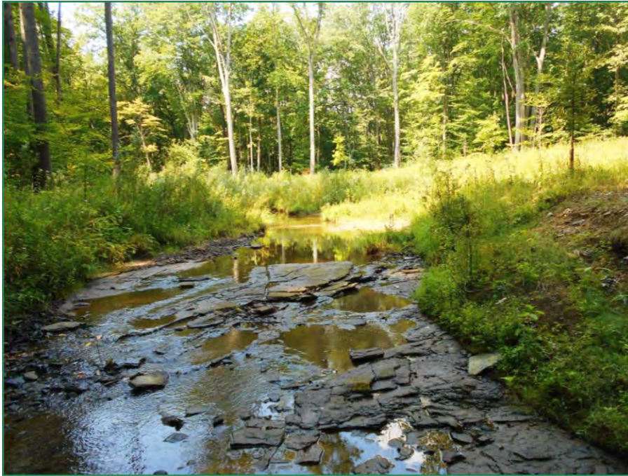
Photograph 1 (August 31, 2015). The eastern limit of the relocated stream channel looking upstream toward the western limit.
