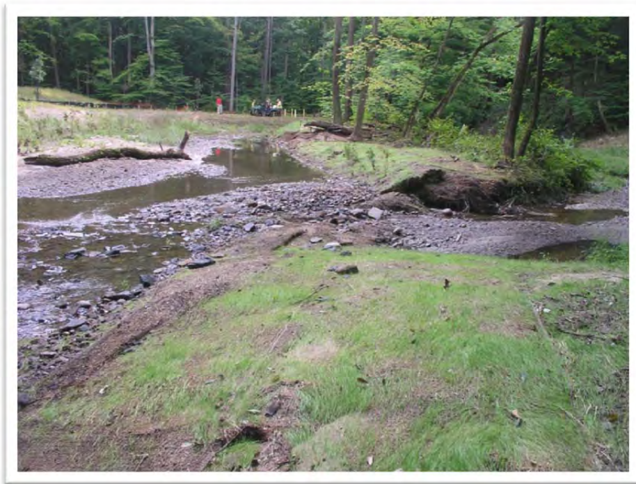
Photograph 5 (July 2, 2013) As can be seen to the right of this photograph, the original channel has been modified so that it does not have through flow, thereby functioning as an oxbow. The relocated channel is to the left.
