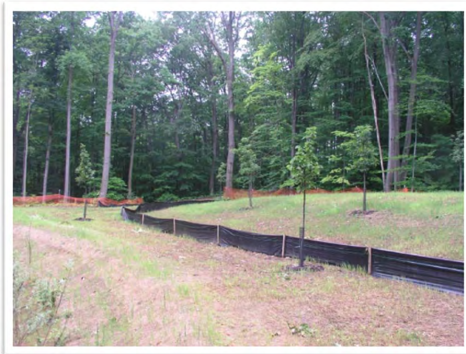
Photograph 1 (August 13, 2013) The open area adjacent to the relocated channel has been seeded and planted with young trees.
