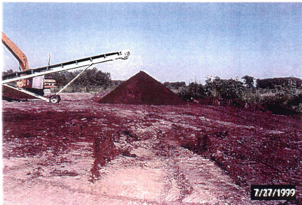
STOCKPILE OF SIFTED SOIL AWAITING EXPLOSIVES AND METALS FIELD SCREENING RESULTS
