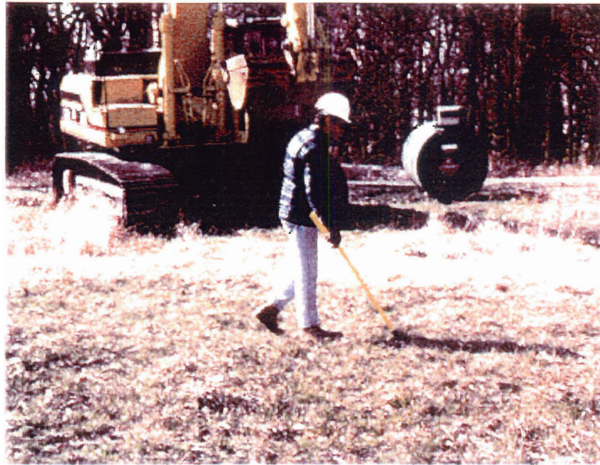
SURFACE SWEEP OF AREA OF CONCERN (AOC) USING SCHONSTEDT
