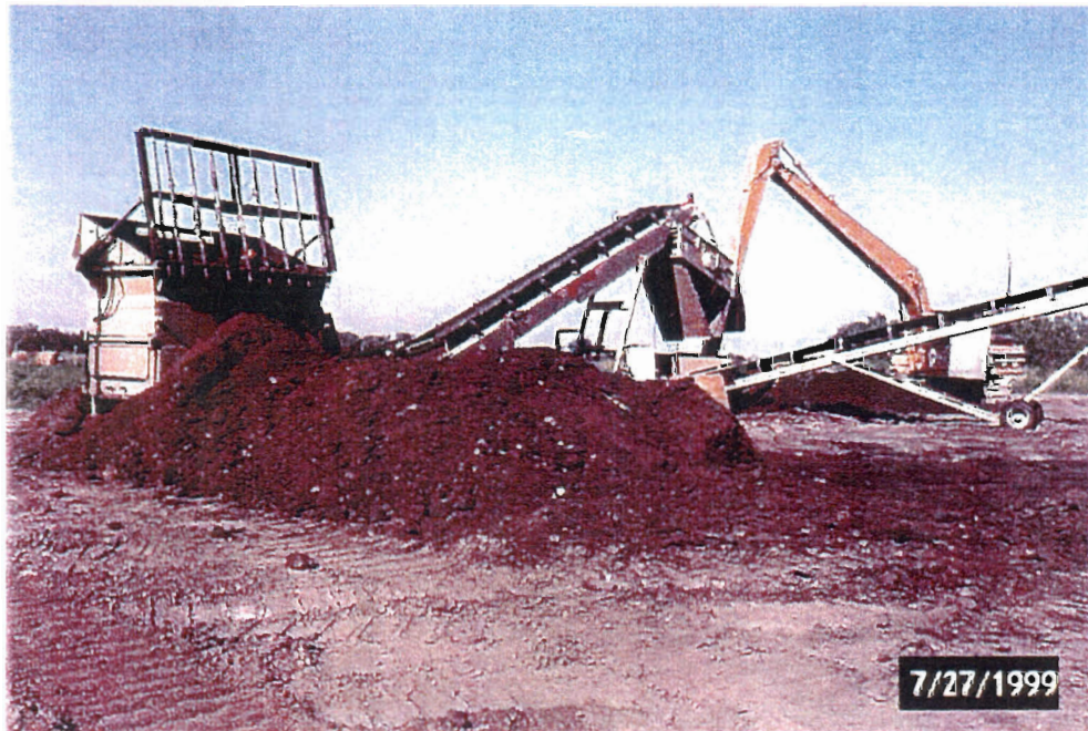
EXCAVATED SOIL BEING LOADED BY THE EXCAVATOR INTO THE SIFTER
