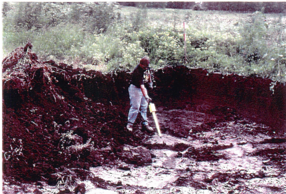
FINAL CLEARANCE OF GRIDS BY UXO PERSONNEL BEFORE BACKFILLING
