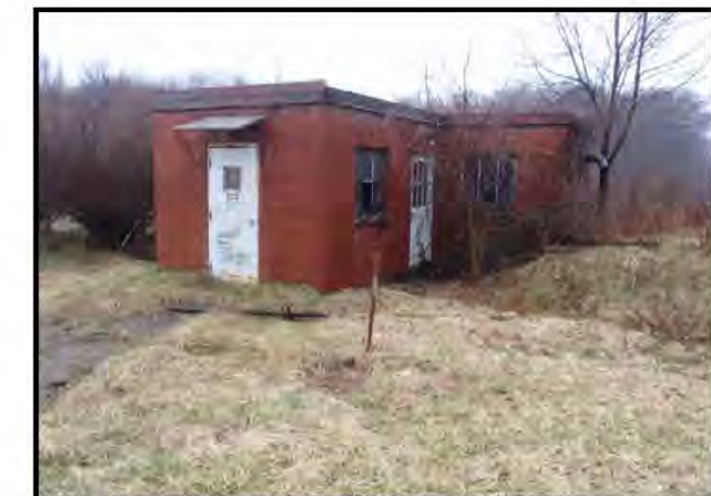
GEORGE ROAD SEWAGE TREATMENT PLANT MAIN BUILDING
