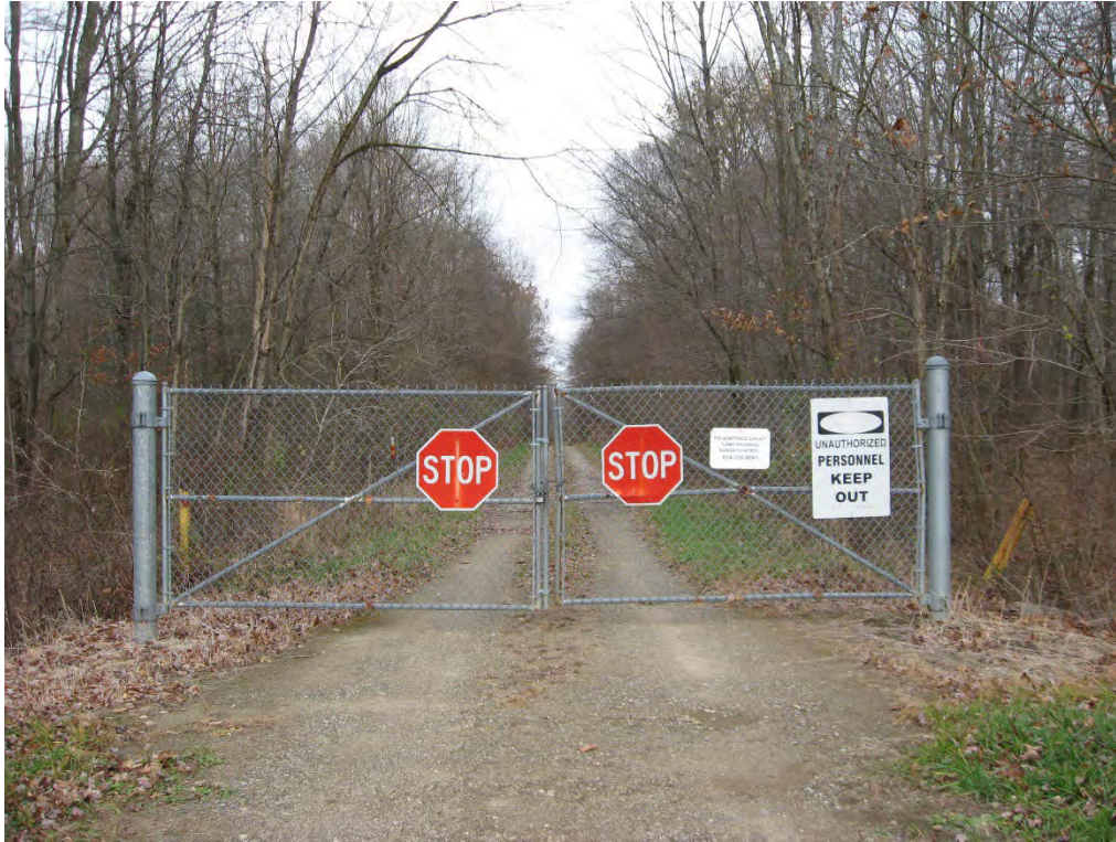
C1. Main gate at Open Demolition Area #2.
