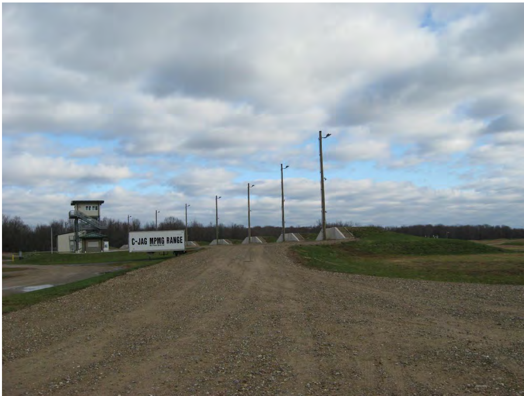
D4. Winklepeck Burning Grounds, looking north from the western portion of the site.
