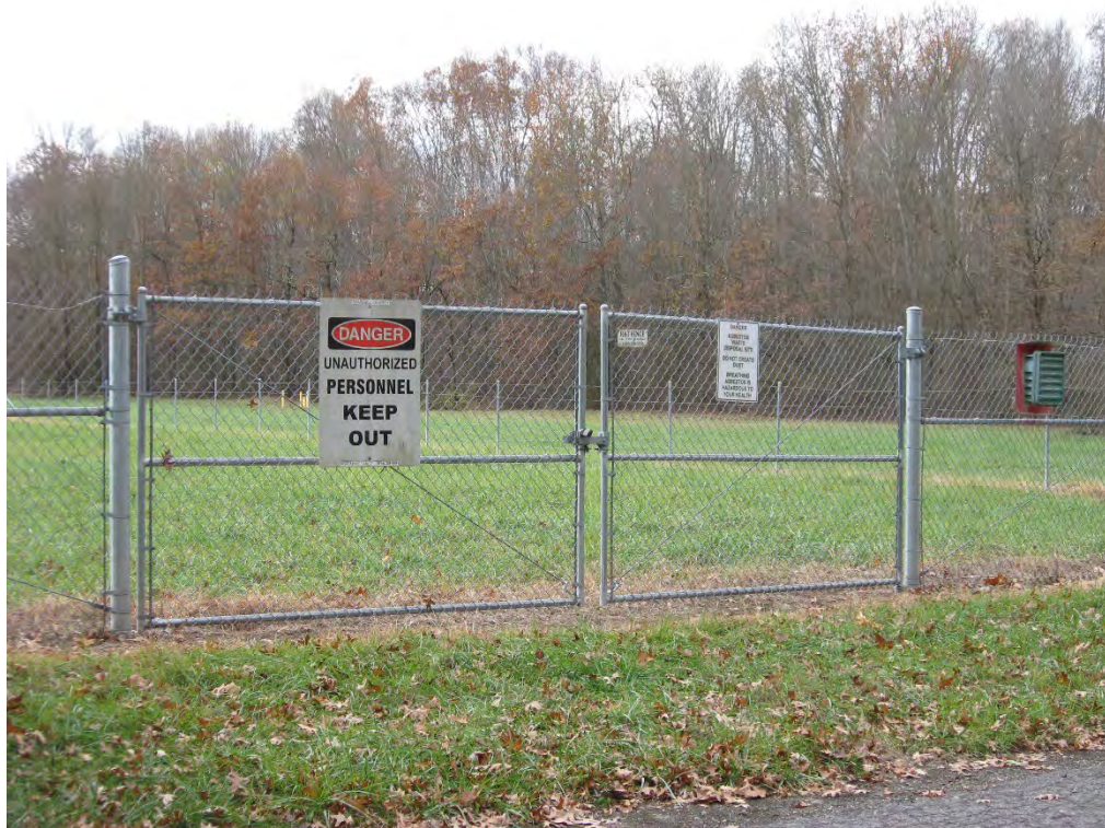
B1. Northwest gate at Ramsdell Quarry Landfill.
