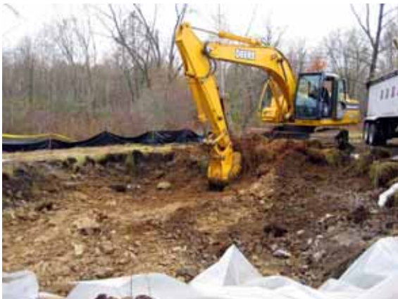
Photograph 4-3. Phase I Excavation of Pile N
