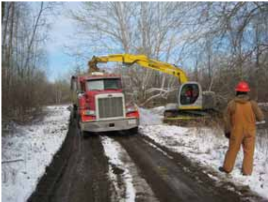
Photograph 4-1. Phase I Excavation of Pile M
