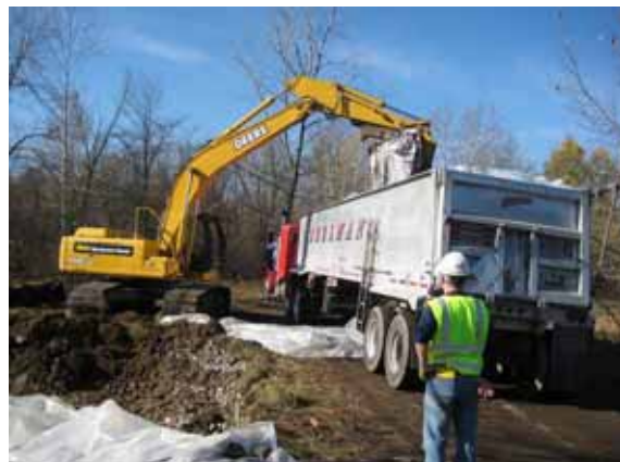
Photograph 4-4. Truck Loading at Pile N
