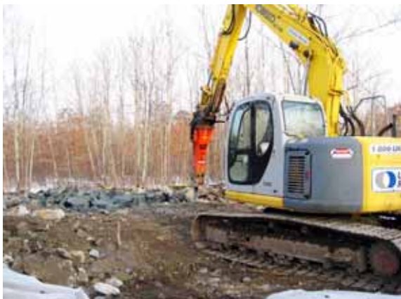
Photograph 4-5. Breaking Up of Concrete at Pile M
