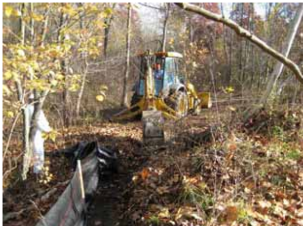
Photograph 3-3. Installation of Silt Fencing
