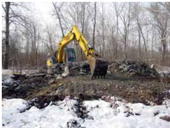
Photograph 4-6. Excavation of Soil and Concrete Aggregate at Pile M
