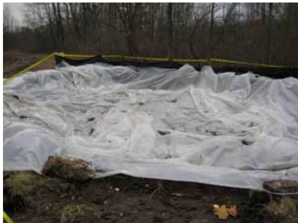
Photograph 3-4. Nightly Cover of Pile N
