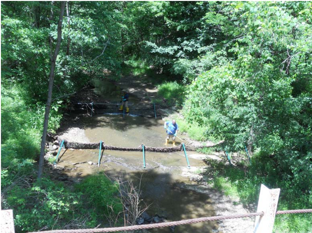
PICTURE SHOWING UXO TECHNICIANS REMOVING DEBRIS FROM BARRIER.
