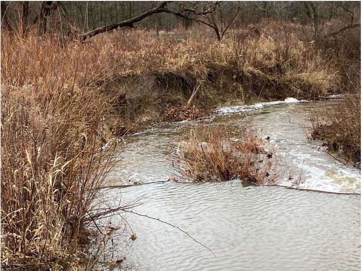
Area of Erosion Down Stream of Beaver Dam
