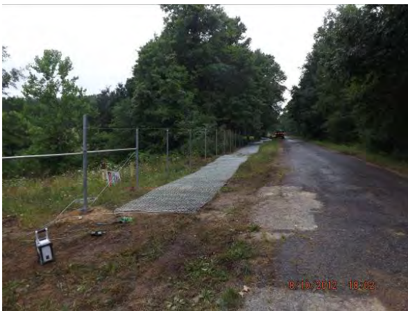
Photograph 5-3. Posts Installed for Chain Link Fence
