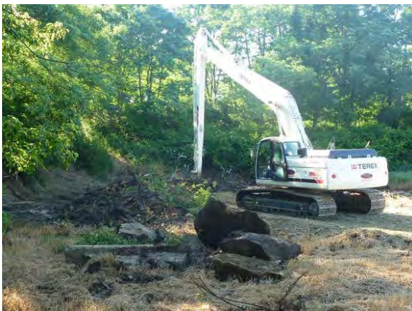
Photograph 3-5. Encountered Construction Debris
