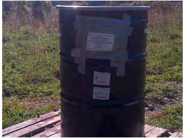
Photograph 5-10. Containerization of an Estimated 200 lbs of ACM
