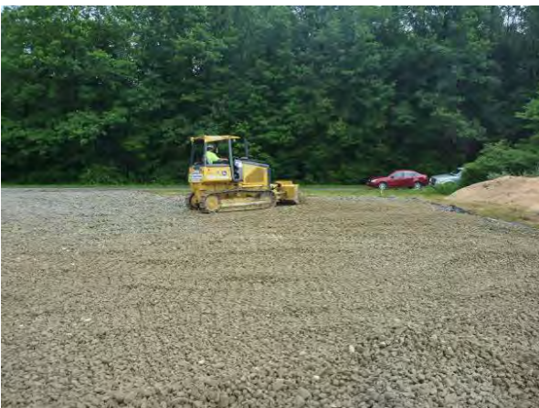
Photograph 3-1. Installation of Equipment Staging Area
