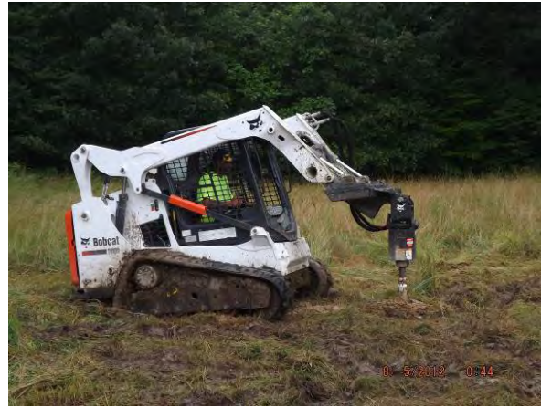
Photograph 5-2. Augering Post Holes
