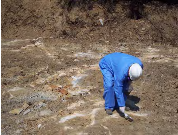
Photograph 3-9. Soil Sampling After Excavation of Removal Area Containing ACM
