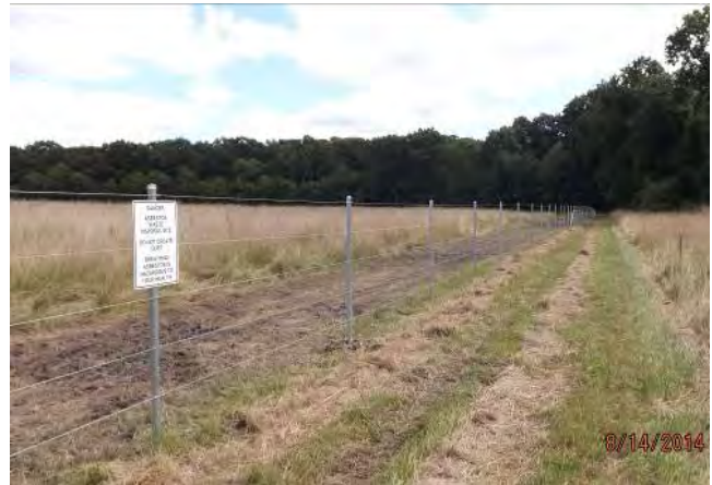
Photograph 5-6. Completed High Tensile Wire Fence
