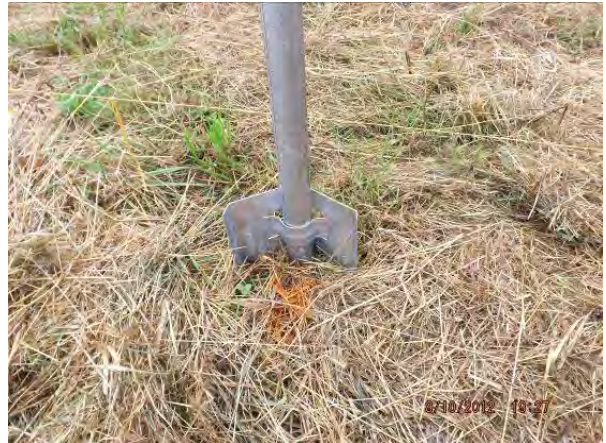
Photograph 5-8. Tubular Post Anchors
