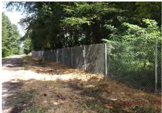
Photograph 5-4. Installed Chain Link Fence
