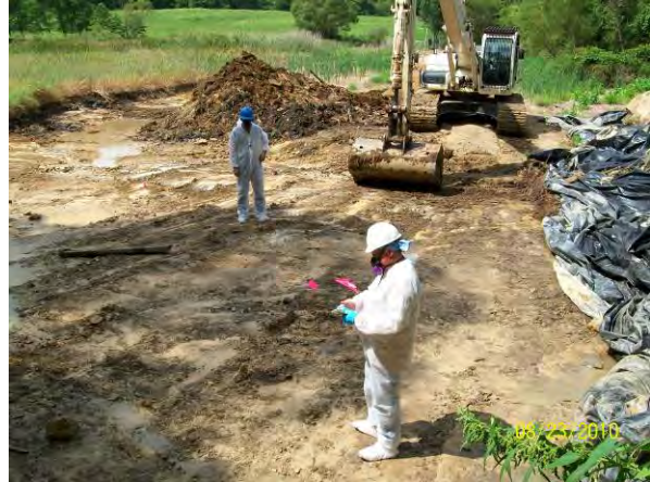
Photograph 3-10. Inspection of Removal Area During Excavation Activities
