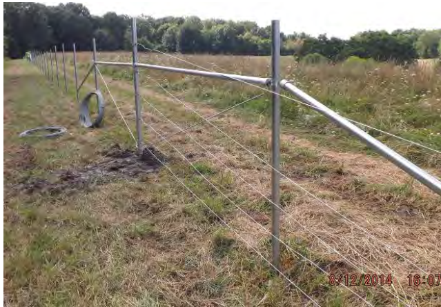
Photograph 5-5. Terminal Posts in High Tensile Wire Fence
