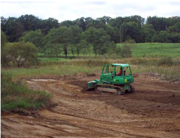
Photograph 3-11. Grading Topsoil During Site Restoration Activities
