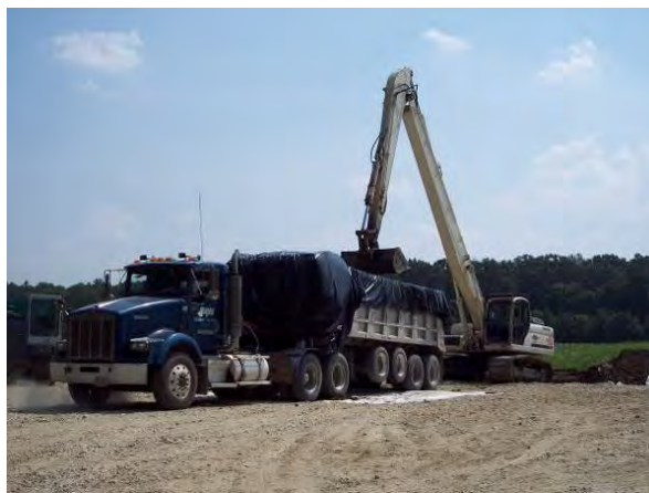
Photograph 3-8. Loading Contaminated Soil into On-Road Haul Truck
