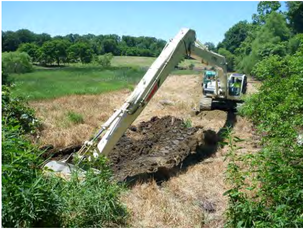
Photograph 3-3. Initial Excavation at Northeast Corner of Quarry Bottom
