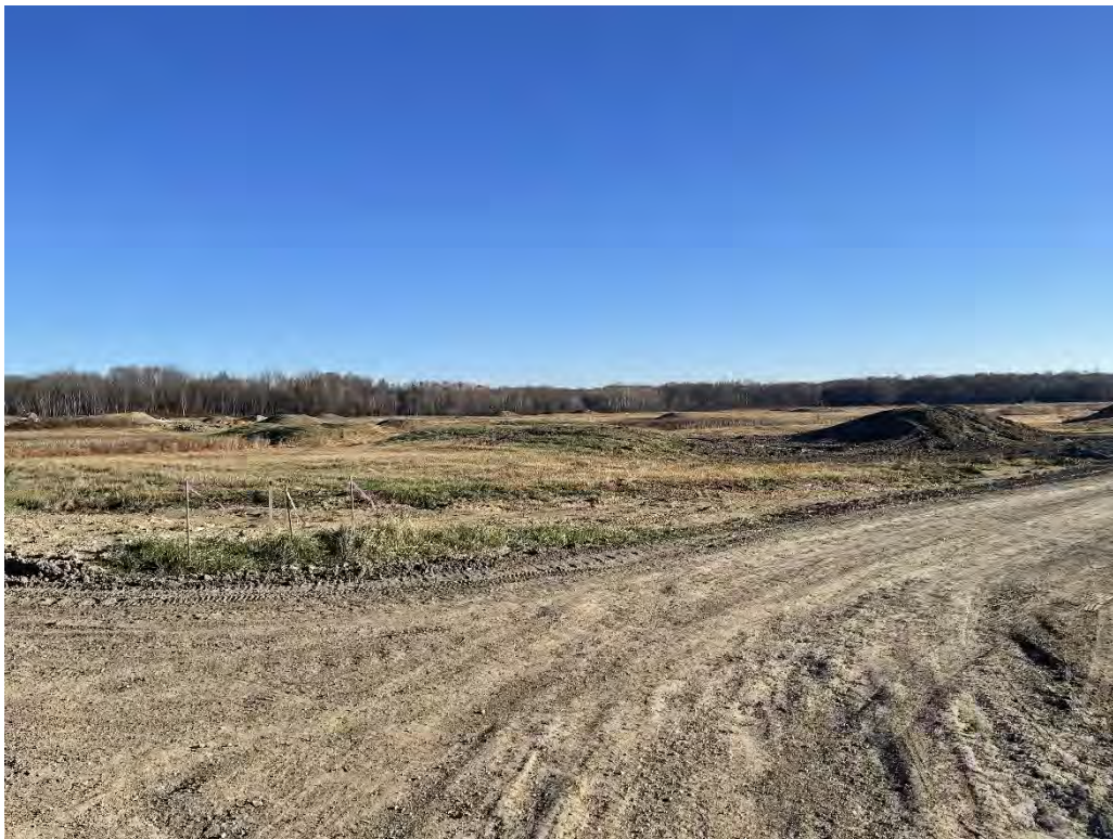
Winklepeck Burning Grounds, looking northeast from the eastern portion of the site.
