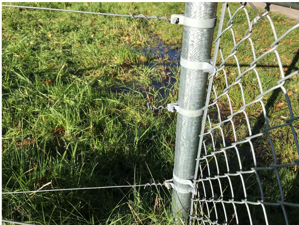
Broken wire of 5-wire tensile fence, northwest corner.
