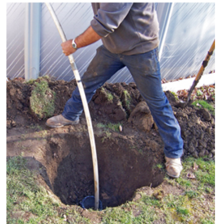
Pressure grouting – early stage.
