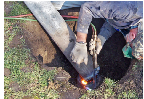
Cutting off the casing.
