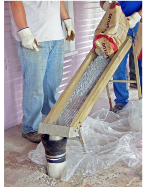
Pouring coarse grade bentonite over mesh screen to filter out fine particles.
