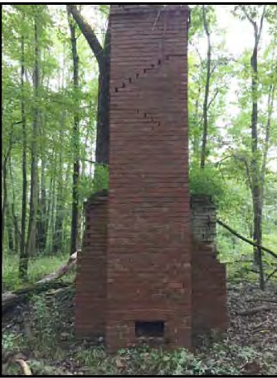
FACING INCINERATOR LOOKING NORTH
